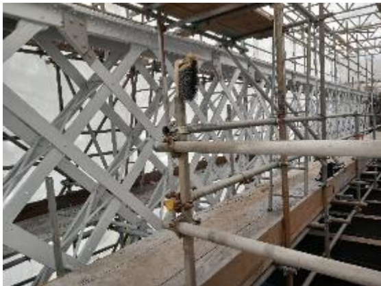
Steel splice Repairs
