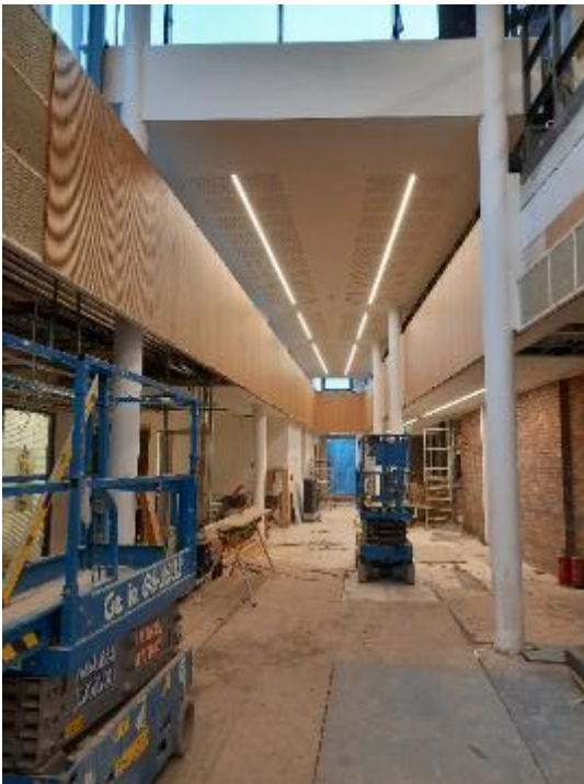
Acoustic Panels White Oak installation (Polished concrete floor with protective covering)
