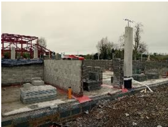
Blockwork and Columns commencement
