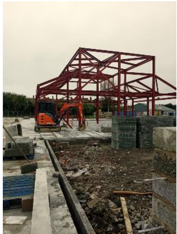
Steel Portal Frame to General Purpose Hall
