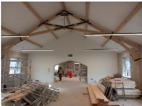
Block C Internal Fit out
