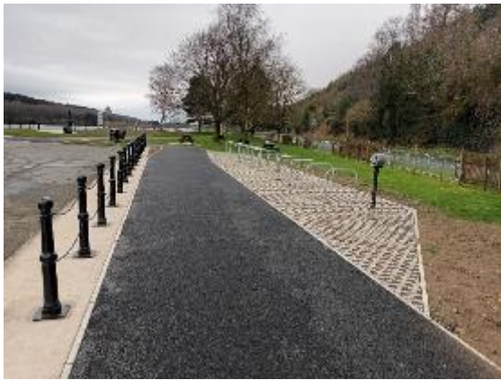
Works Complete in Victoria Lock in NI
