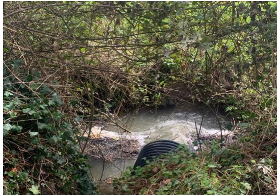
Drainage Remediation- R166
