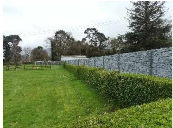
Accommodation Works Precast Wall
