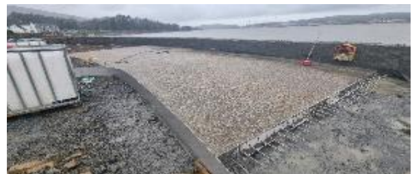
Concrete exposed aggregate footpath Installation
