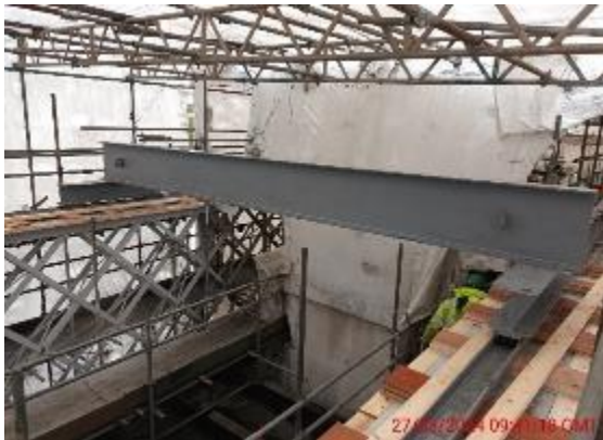
Beam replacement gantry support assembly
