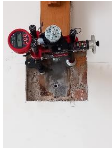
Block B Corbel Pull Test to 2.5 Tonnes
