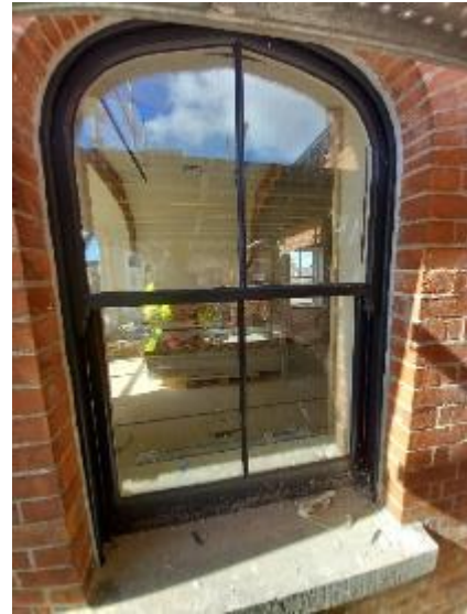
Window sealing sample Block B Council Chamber
