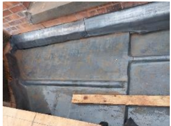
Lead Roof installation Bay Window Block B
