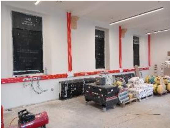
Block C Comms fit out
