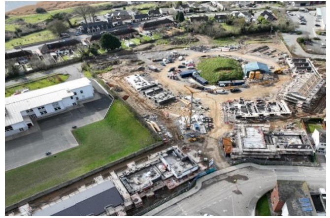
New Housing Scheme under construction at Boice Court, Drogheda.
