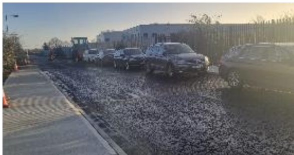
New carriageway with footpaths
