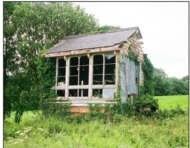
Fig 5.10 Signal Cabin at Newbliss.
