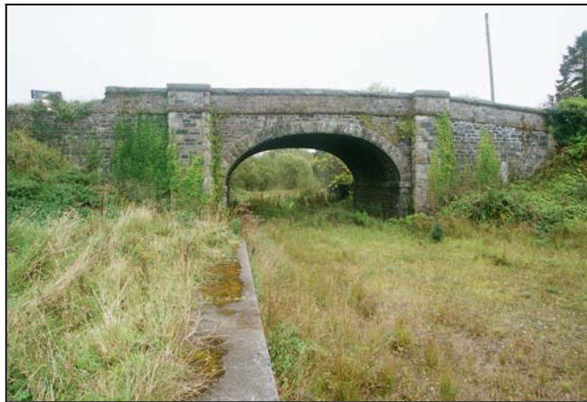
Fig 5.17 Semi-elliptical arched road bridge over line just east of Newbliss Station (03726).
