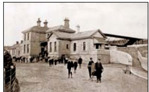
Fig 5.2 Clones Station, opened in 1858.
