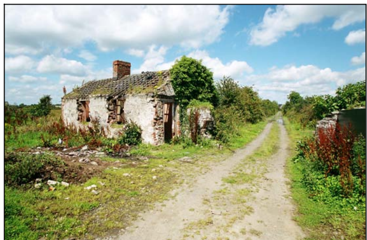
Fig 10.11 Crossing house and track bed, Marsh North townland (08206).
