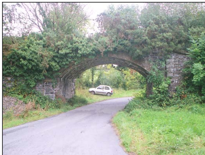
Fig 8.5 Rail/road bridge south of Rockcorry (06205).
