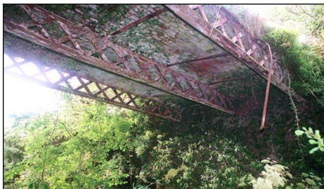
Fig 8.6 Detail of lattice girder bridge, Lisgillan townland (06113).
