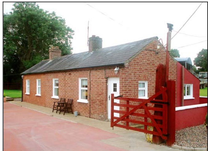
Fig 9.14 Level crossing house at Faulkland Crossing, north-east of Monaghan (07217).
