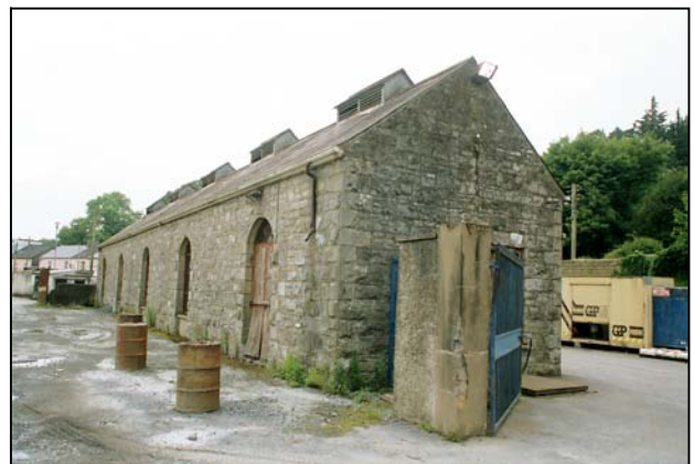
Fig 9.7 Offices and workshops at the Ulster Yard, Clones (07430).
