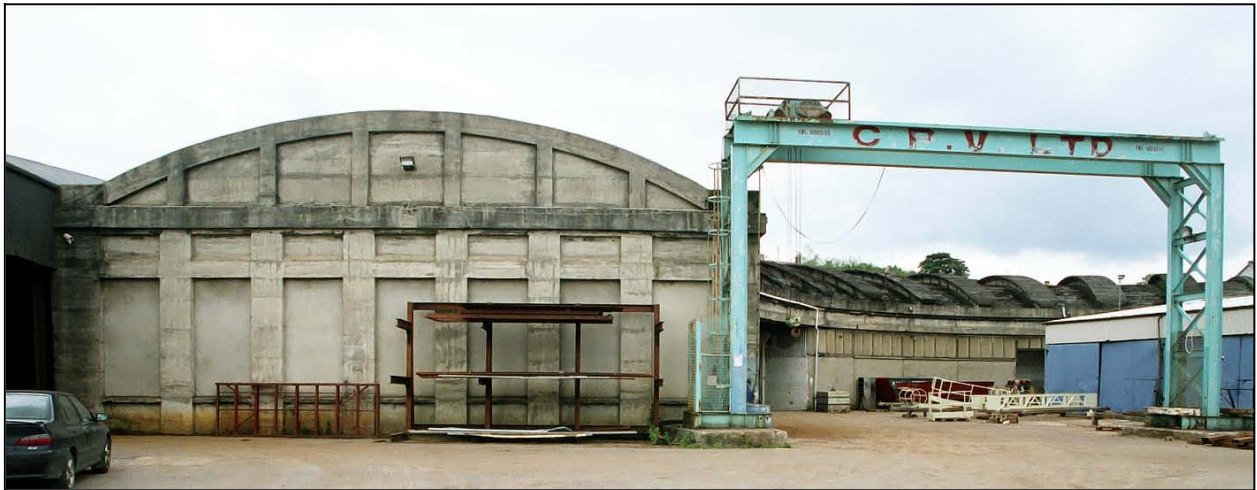
Fig 5.11 The reinforced-concrete engine shed at Clones Station.
