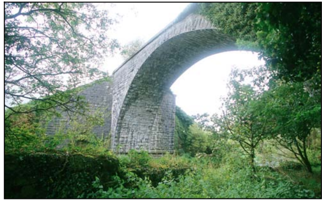
Fig 5.14 Rail bridge over the Finn River near Anlore.
