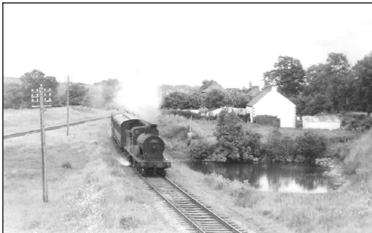
Fig 9.3 Train en route to Cavan, just after leaving divergence with Enniskillen line (C. Friel Collection/ R.M. Arnold).
