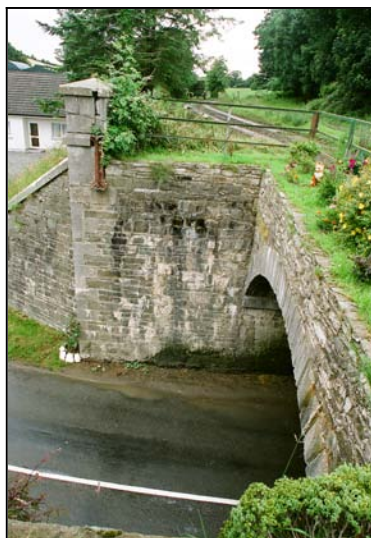
Fig 6.6 Rail bridge at Inniskeen on the Dundalk-Enniskillen line, widened to accommodate Carrickmacross branch.
