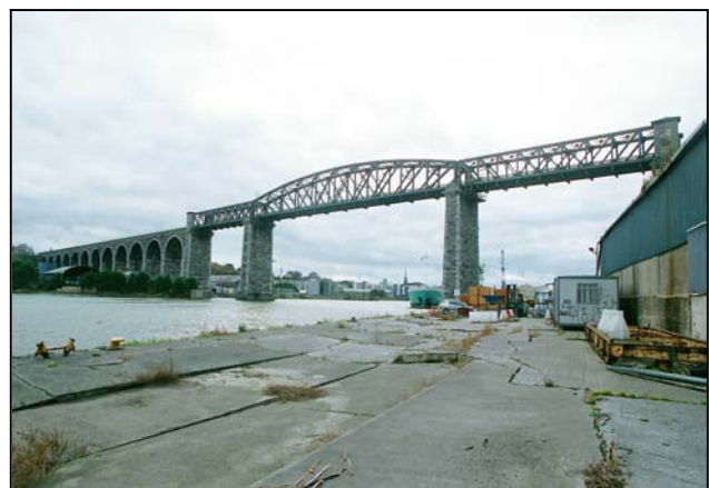
Fig 3.3 Boyne Viaduct with replacement steel spans.
