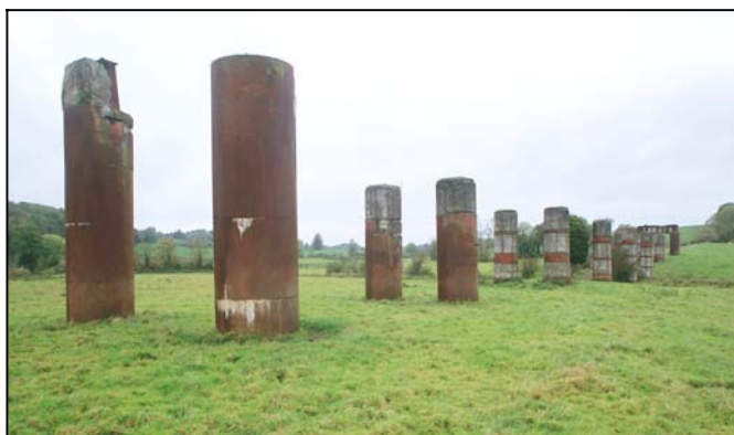
Fig 5.15 Remains of girder beam bridge near Anlore.
