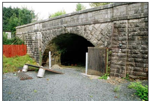
Fig 5.20 Northern portal to tunnel just south of Castleblaney Station (03426).
