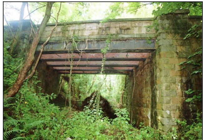
Fig 11.7 Metal beam bridge near Co Armagh border (09314).
