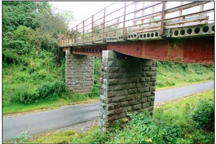
Fig 5.16 Girder accommodation bridge over former track just north of Culloville Station.
