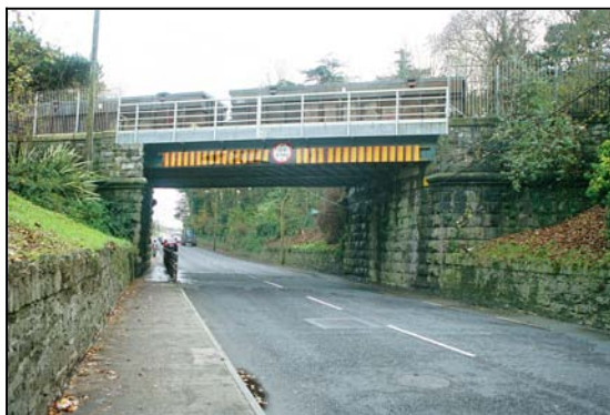
Fig 13.4 Skew plate girder bridge over Dublin Road.
