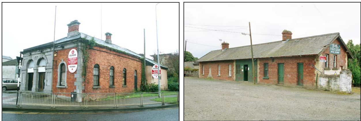
Fig 10.8 Left Quay Street Station, Dundalk. Right Bush Station.
