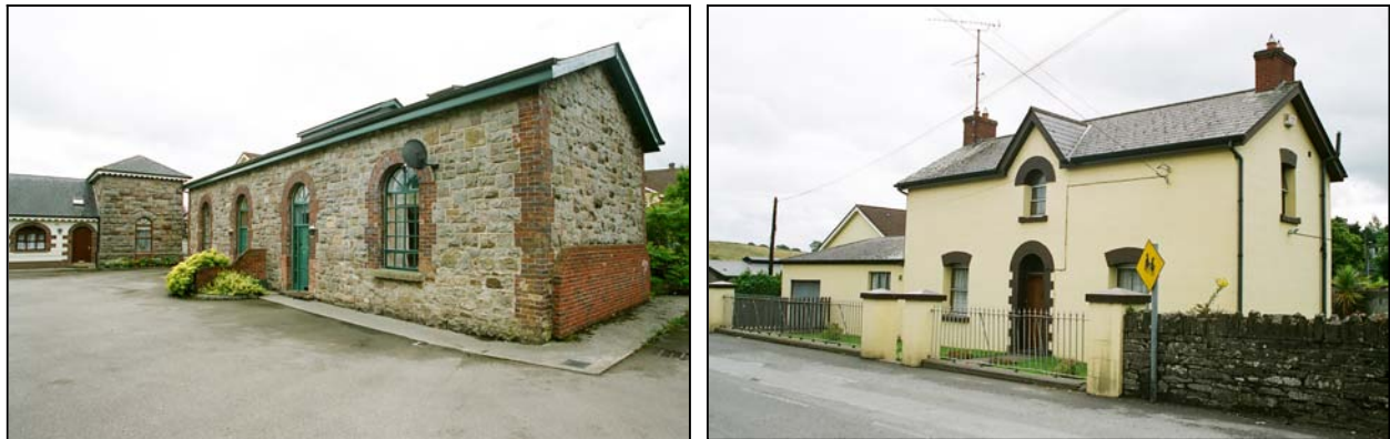
Fig 6.4 Left: Converted engine shed at Carrickmacross. Right: Former station master's house.
