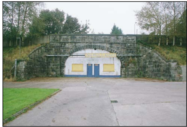
Fig 9.12 Road bridge east of Smithborough Station (07333).
