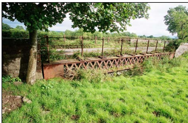
Fig 9.11 Partly buried lattice girder bridge near Stone Bridge (07417).
