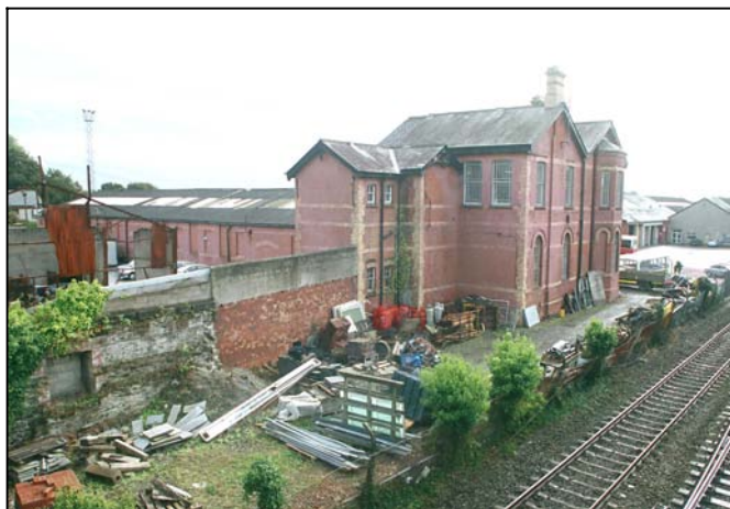
Fig 3.6 The former General Stores at the GNR Works.
