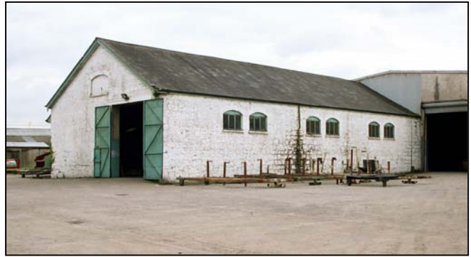
Fig 5.8 Goods shed at Clones.
