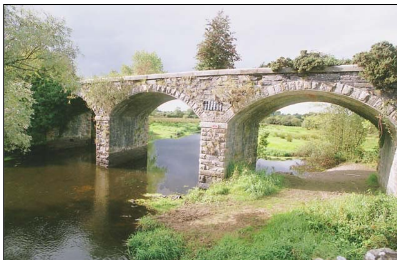
Fig 8.4 Bridge over River Finn near at Ballynascarva.
