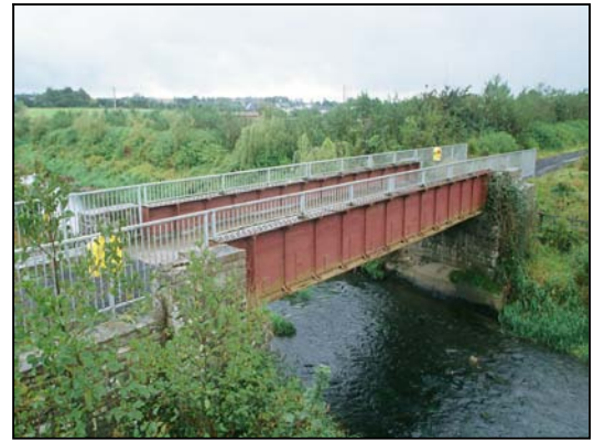
Fig 4.6 Rail bridge over the Dee.
