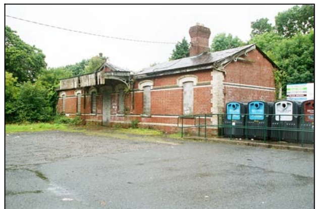
Fig 3.4 Dunleer station building.
