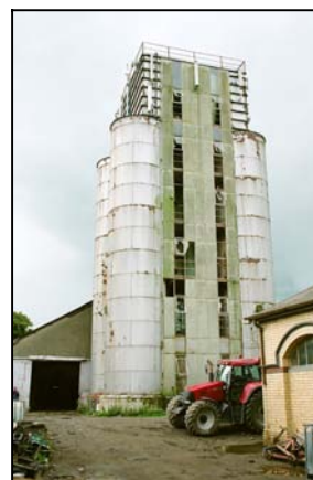
Fig 4.5 Ardee station building (left) and grain silos (right).
