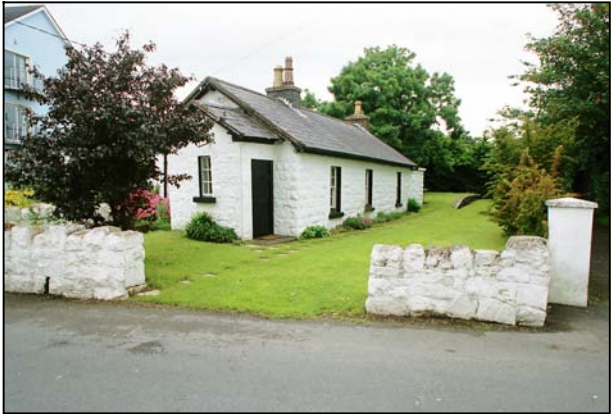
Fig 11.9 Level crossing house, Omeath (09250).
