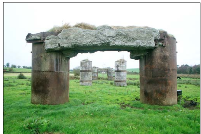
Fig 5.13 Remains of girder beam bridge over Ulster Canal near Clones.
