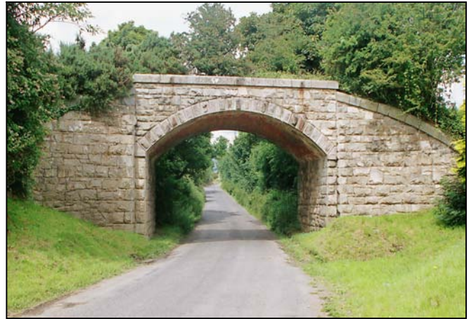
Fig 10.9 Rail bridge over road, Piedmont (08312).
