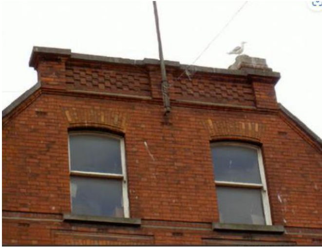
Figure 3 – shows the parapet wall and brick detailing on the front elevation.
