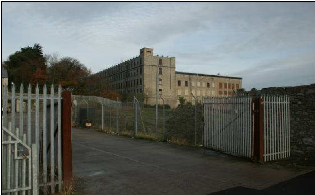
Plate 78: Bessbrook former mill, Co. Armagh (No. 36)
