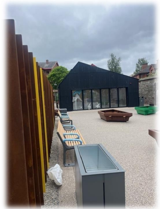
The new Visionary Solutions at Dundalk are almost complete.
