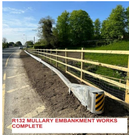
R132 Mullary Embankment Works Complete
