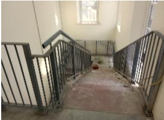
Block E, fire escape stairs.
