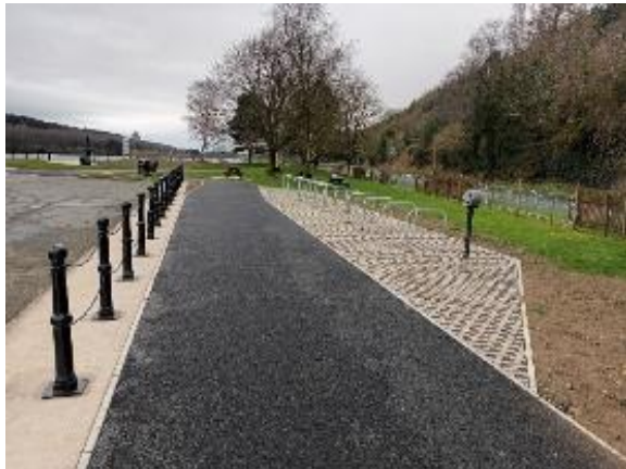
Works Complete in Victoria Lock in NI
