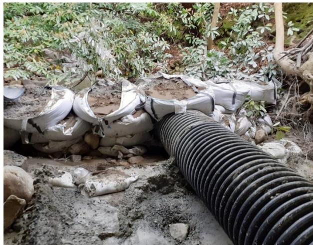
Works taking place at Connolly bridge, North Louth
