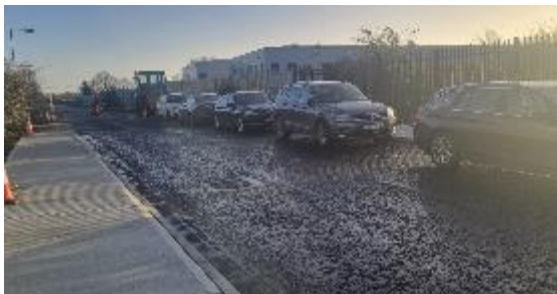
New carriageway with footpaths
