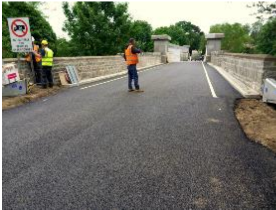
Final Works North Side of the Bridge
