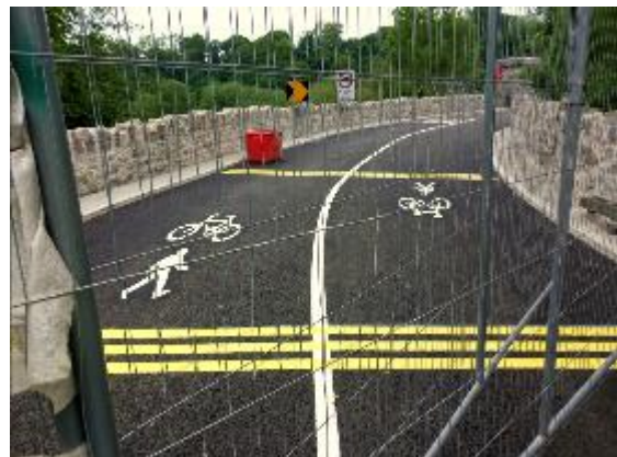
South Side Road Marking prior to opening
