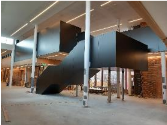
Main Stair Case Final Lacquering
