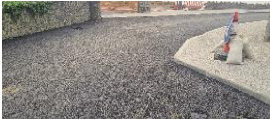
New Road Surfacing Shore Rd.
