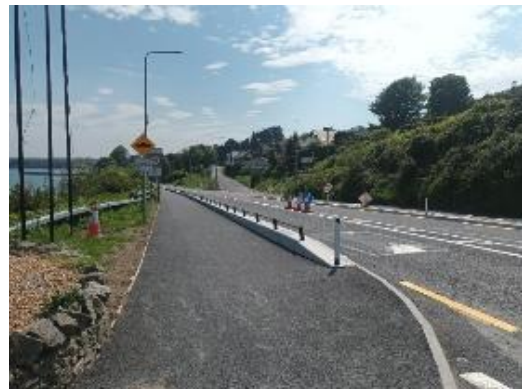
Section of completed footway at Carlingford Marina.
