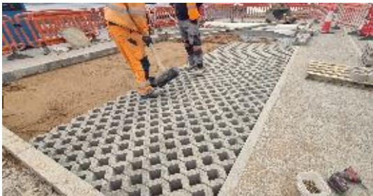
New "Grasscrete" sets being laid in pier area.
