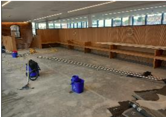
Fixed Seating at Mezzanine Floor commenced.
