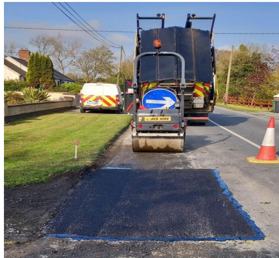
Figure 1LS-6292-0 Tinure JCB PRO repair
