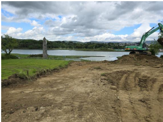
Earthworks Cut commencing.
