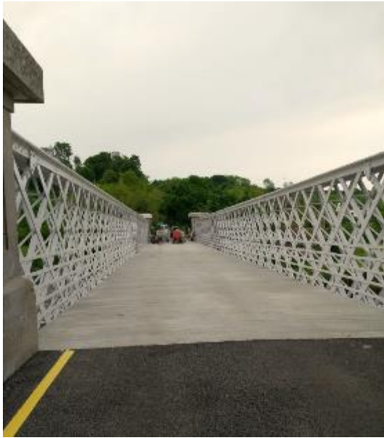
Completed Bridge Deck
