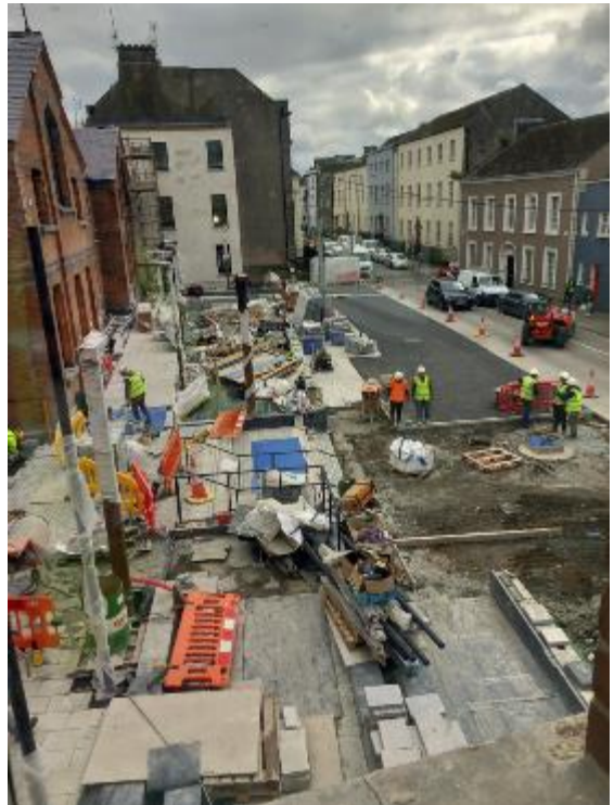
Block B and N (Main entrance) and ongoing external works
