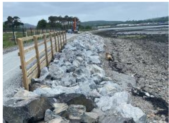
Rock Armor Repair
