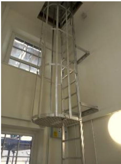
Roof Access Ladder.
