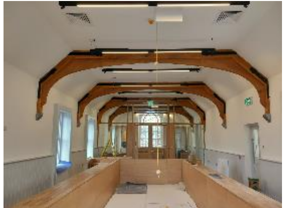
Council Chamber fixed furniture installation
