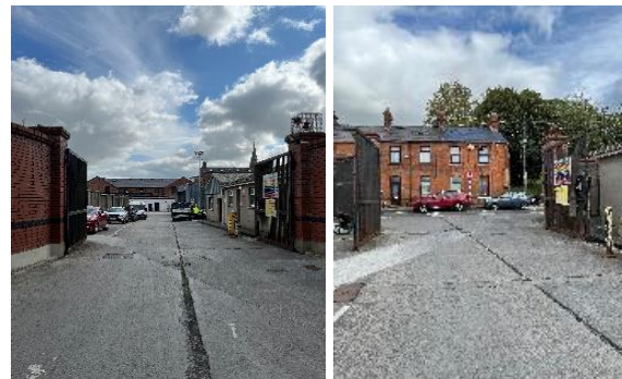
Machinery Yard Entrance to the Council's Drogheda Office
