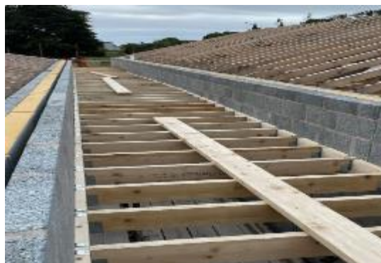
Roof Trusses installation
