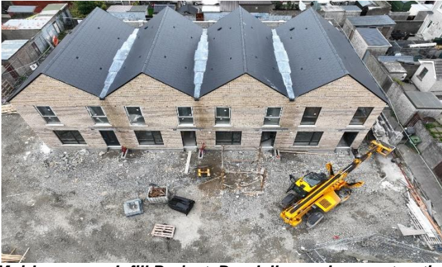
Muirhevnamor Infill Project, Dundalk – under construction
