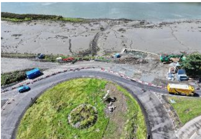
Culvert Works Northern Approach.
