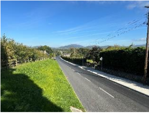
Finished works south of Castletown Cross
