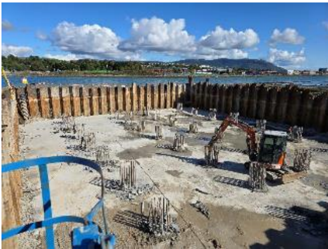
Piling Works Southern Abutment
