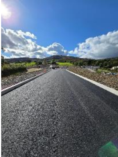
Roadworks Southern Approach.
