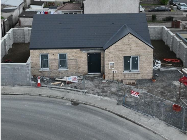
Muirhevnamor Infill Project, Dundalk – under construction
