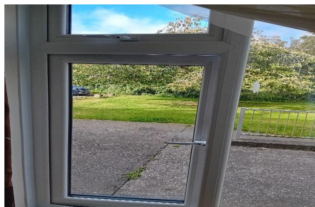
New Windows fitted in Drogheda in September, funded by a HOPS
