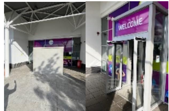
Improvements at the front entrance at Dundalk Leisure Centre
