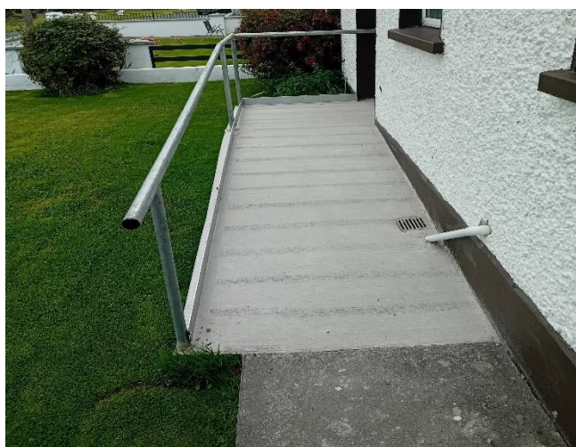
Access ramp in Dunleer completed in September, part-funded by a HAG
