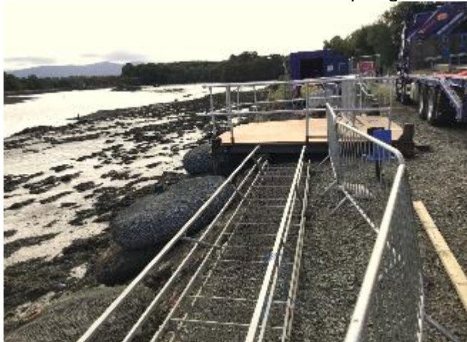
First Section of Boardwalk substructure
