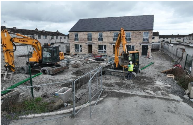
Muirhevnamor Infill Project, Dundalk – under construction
