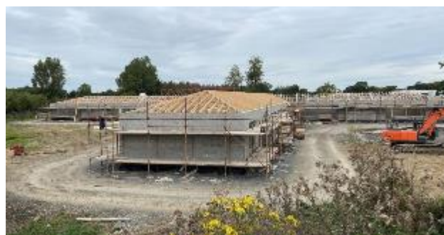
Overall site Progress
