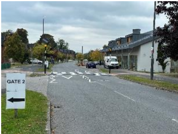
New Controlled Crossing in Lis Na Dara
