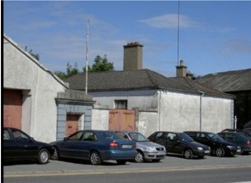
Figures 3: Side elevation of the protected structure, with limited view of the shed structure located to the rear.
