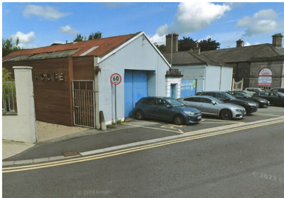
Figure 4: Shows the existing storage shed located to the rear of the protected structure.
