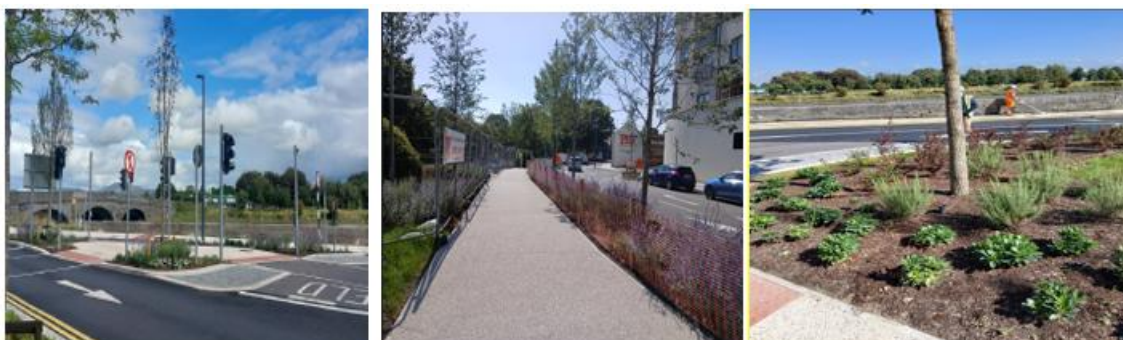
St Nicholas Quarter Phase 1 Public Realm Works
