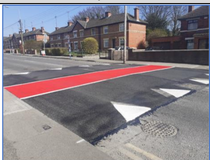
Traffic calming in Drogheda 2025 integrating pedestrian safety
