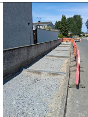
Footpath improvement works.
