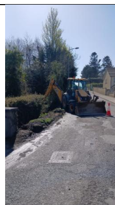
Drainage and Verge works
