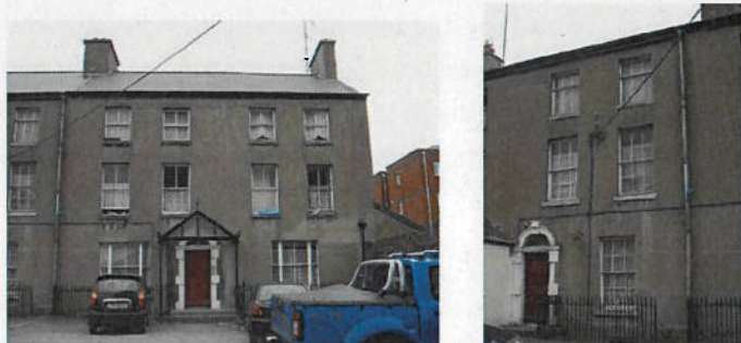
Figure 1: Front Façades - No.'s 1 & 2 Paradise Place
