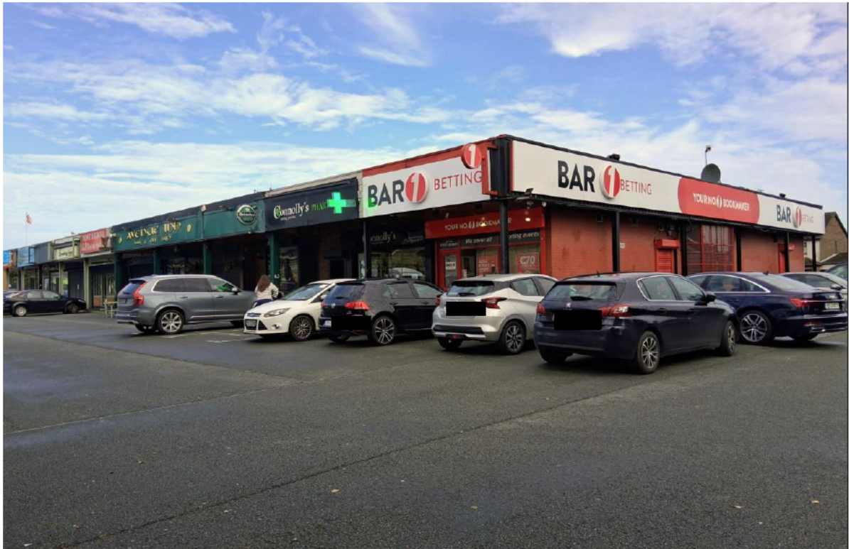
Fig.2: Existing building (taken 25/09/2026.)
