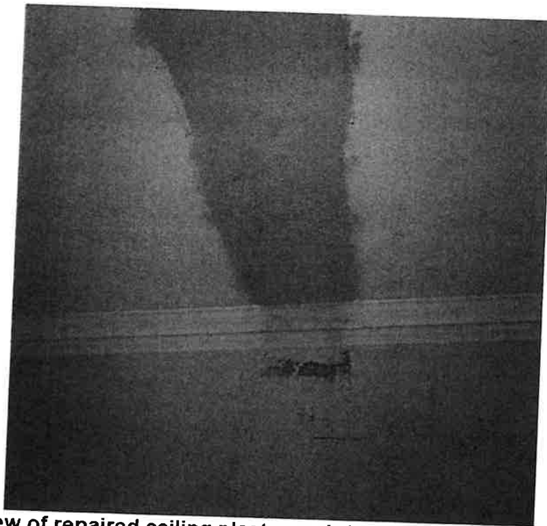
Image 4 – View of repaired ceiling plasterwork (unpainted).
