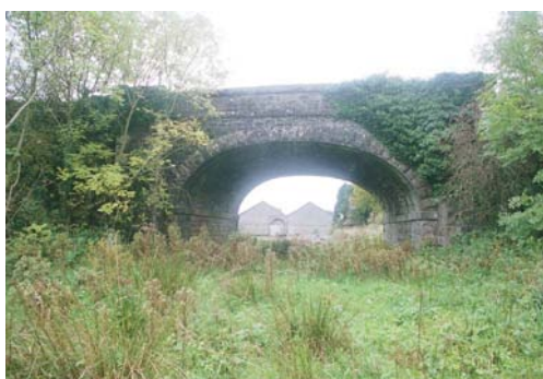
03726_01 FWH 11/10/2007 East elevation. Note Newbliss Station buildings behind.
