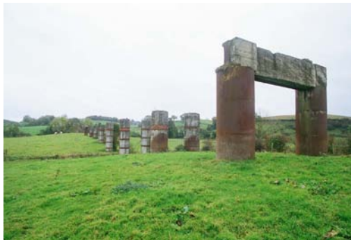
03817_04 FWH 23/10/2007 Viaduct from NW.
