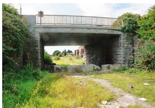
03107_01 FWH 31/07/2007 East elevation of bridge.
