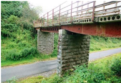
03402_03 FWH 09/08/2007 NW elevation, from west.
