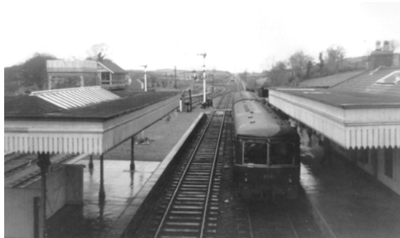
Inniskeen Station, looking west from the footbridge.
