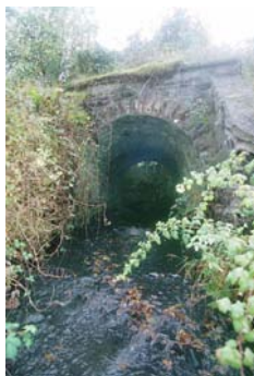
03806_01 FWH 11/10/2007 Upstream (N) elevation.
