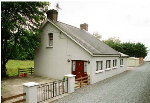
03701_18 FWH 25/06/2007 Station house, from NE.
