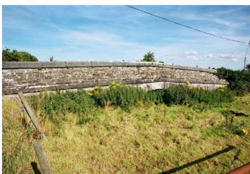
03206_01 FWH 31/07/2007 West elevation of bridge.
