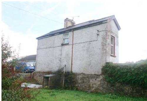
03626_02 FWH 21/09/2007 Level crossing house, from NW.
