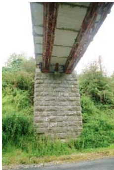
03402_04 FWH 09/08/2007 Looking NE along underside of middle span.
