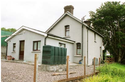
03701_19 FWH 25/06/2007 Station house, from SW.
