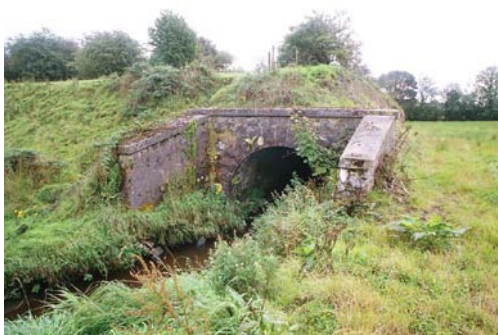
03628_01 FWH 21/09/2007 Bridge from NW.
