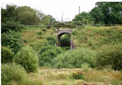
03508_01 FWH 24/07/2007 View of bridge from north.
