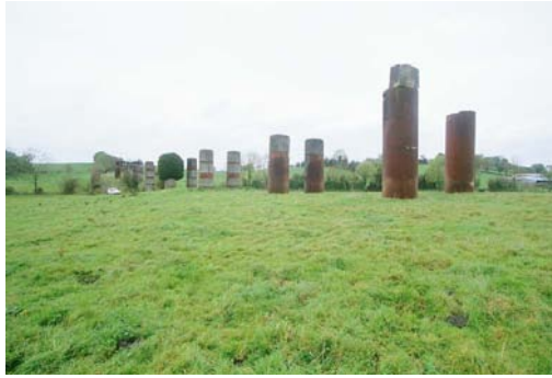
03817_03 FWH 23/10/2007 Viaduct from SE.
