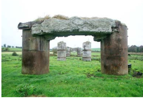
03822_02 FWH 23/10/2007 Looking west from east end of former viaduct.
