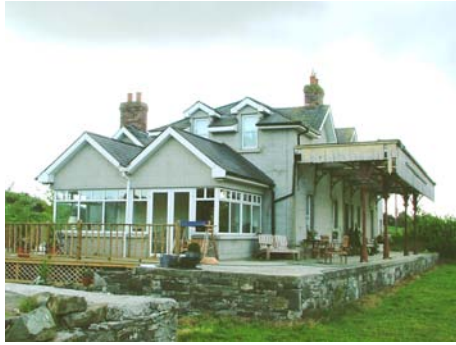
03301_03 AR&R 25/09/2007 West elevation of station building.
