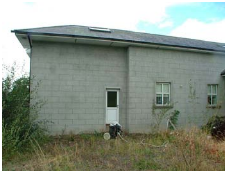
03301_05 AR&R 25/09/2007 East (rear) elevation of station building.
