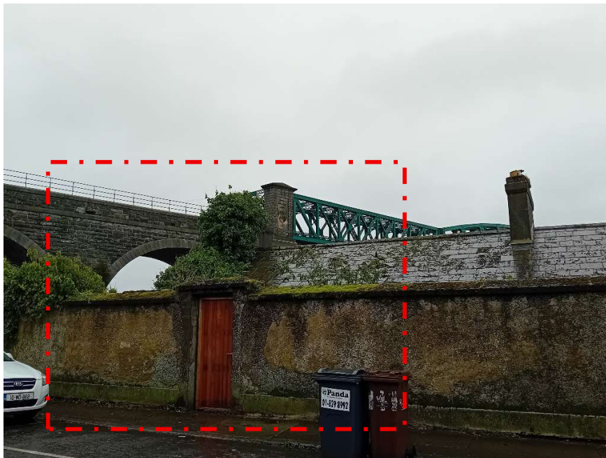
Figure 2 – Shows the structure from Boyne Terrace, Drogheda.
