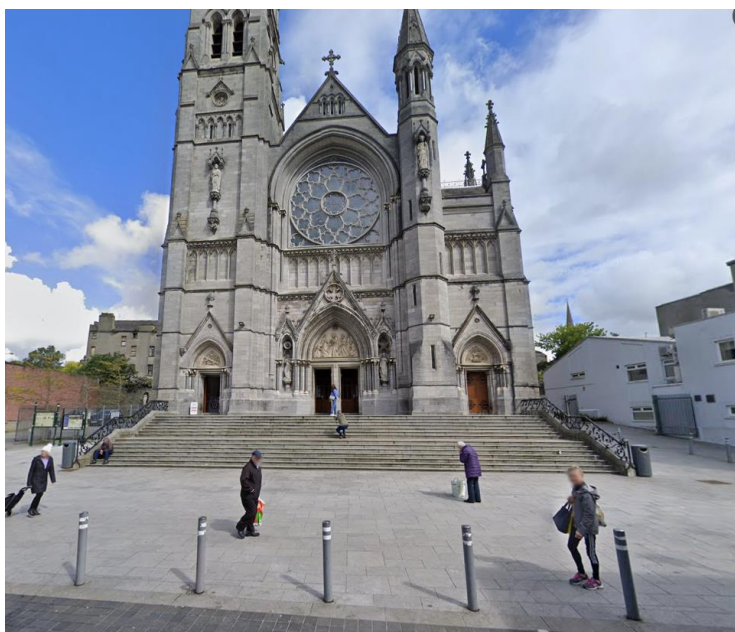
Figure 1: Protected Structure as viewed from West Street
