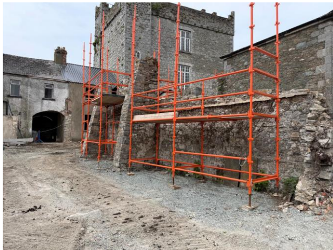
External to Rear – Rebuilding of rubble stone wall
