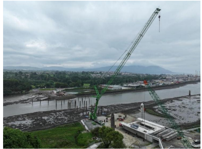
650t Crane for temporary skid beam bracing installation.
