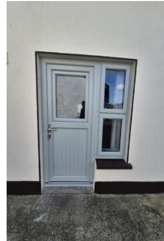
New Door completed in Ardee with funding Provided with a HOP
