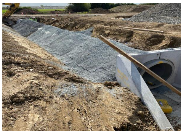
CH300 – 1200mm Culvert
