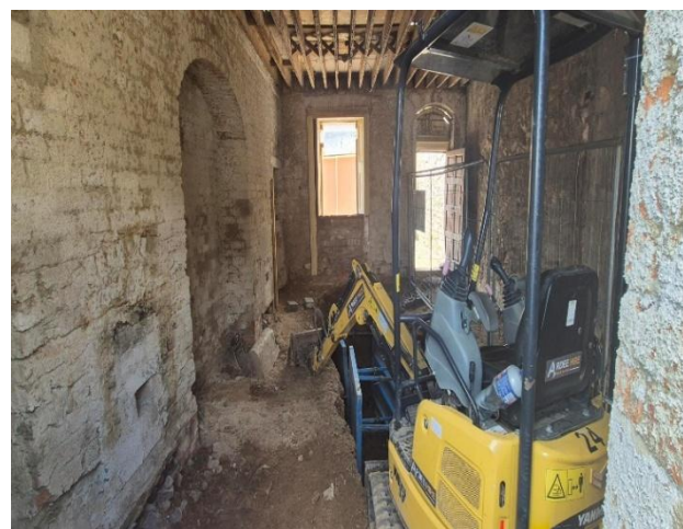
Sub-Floor Drainage Works
