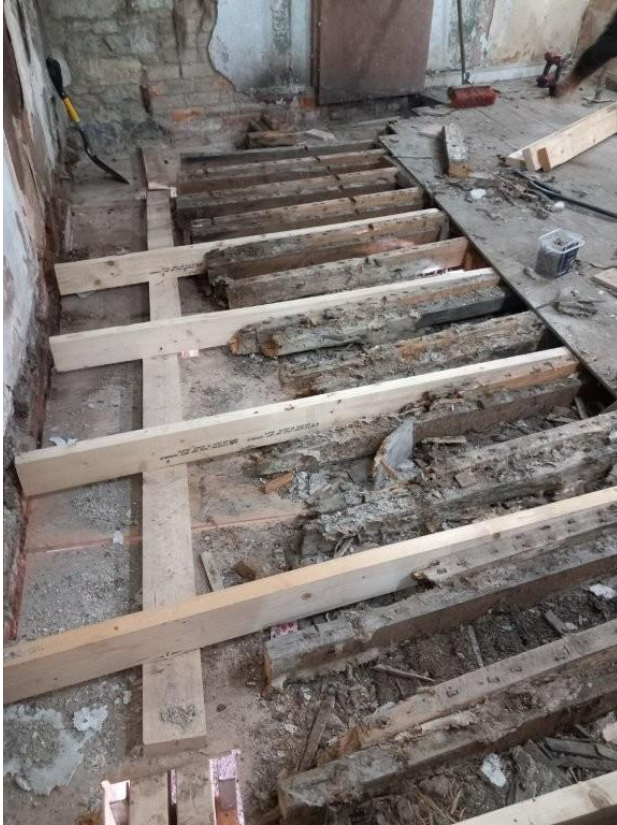
Spliced Repairs to Wooden Joists
