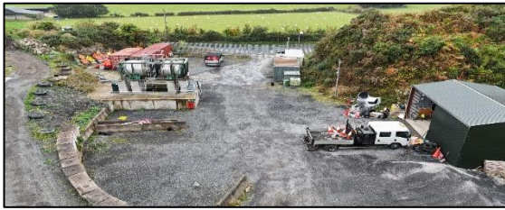
The existing Bush Depot at Ballaverty Millmount Maintenance works
