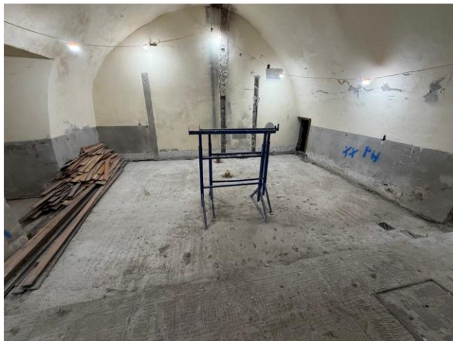
Tower Ground Floor – screed removed
