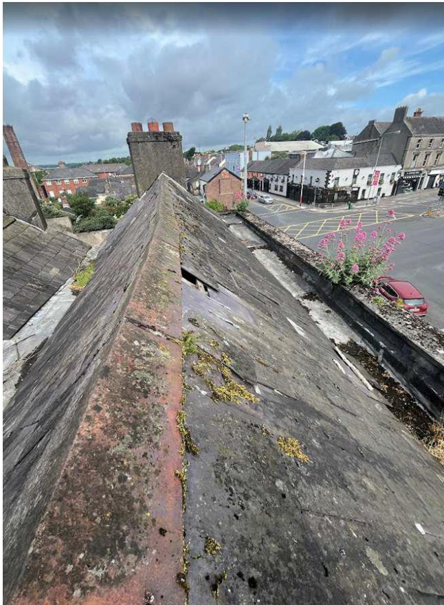
Slipped/Missing Tiles
