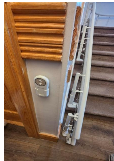
Stairlift completed in Dundalk, with funding provided provided with a MAG
