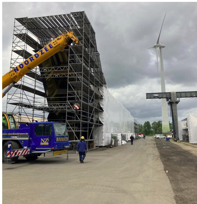
Encapsulation system for the pylon to allow painting
