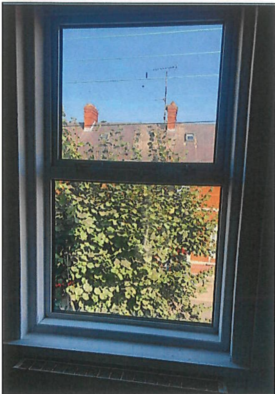
Repairs to existing windows
