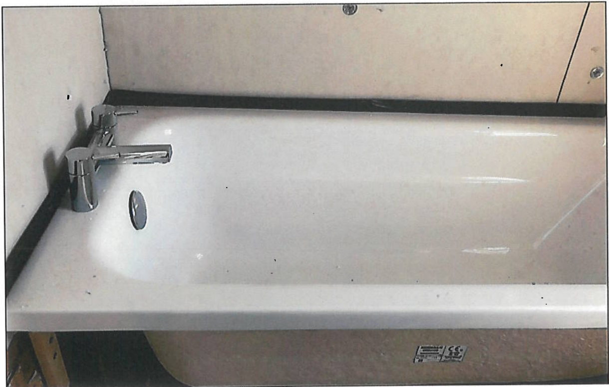
New bath & plumbing
