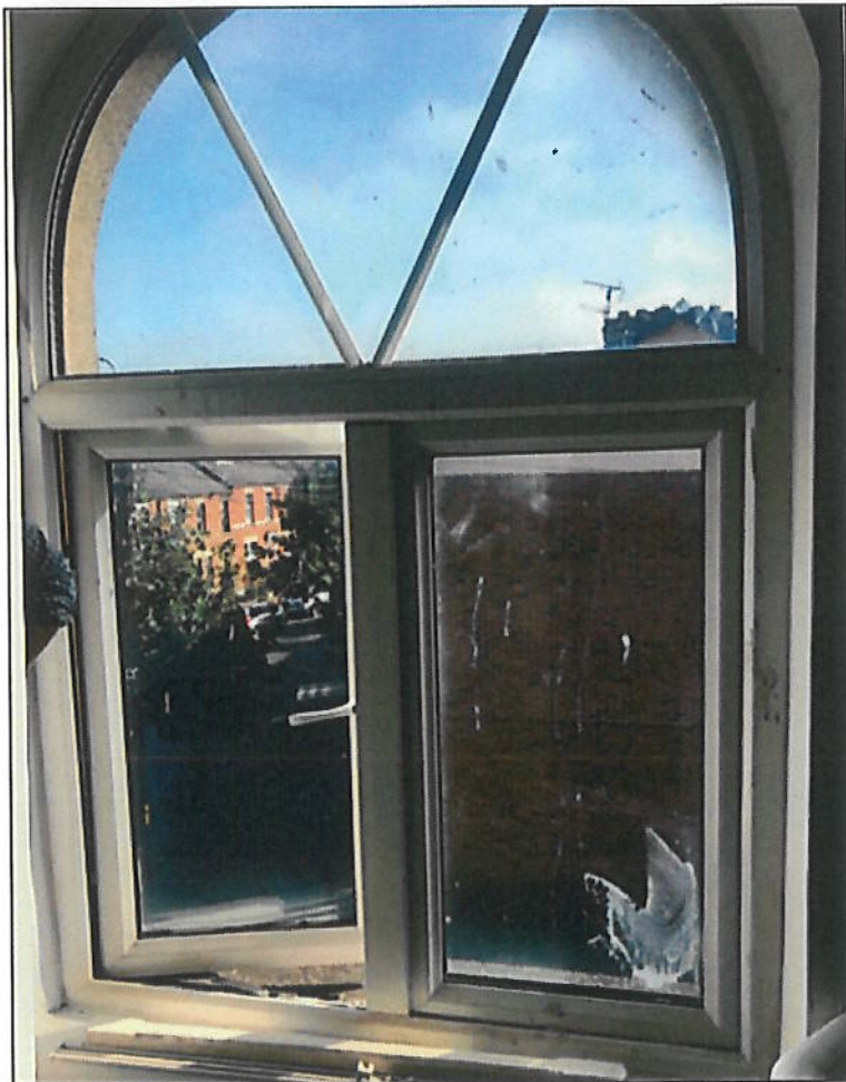
Pvc Window repairs – lieu of wooden windows.
