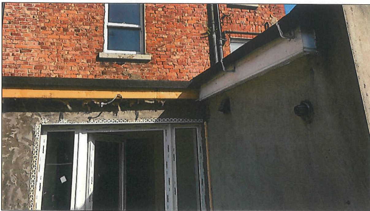
External facade alterations to extension including guttering plastering etc.
