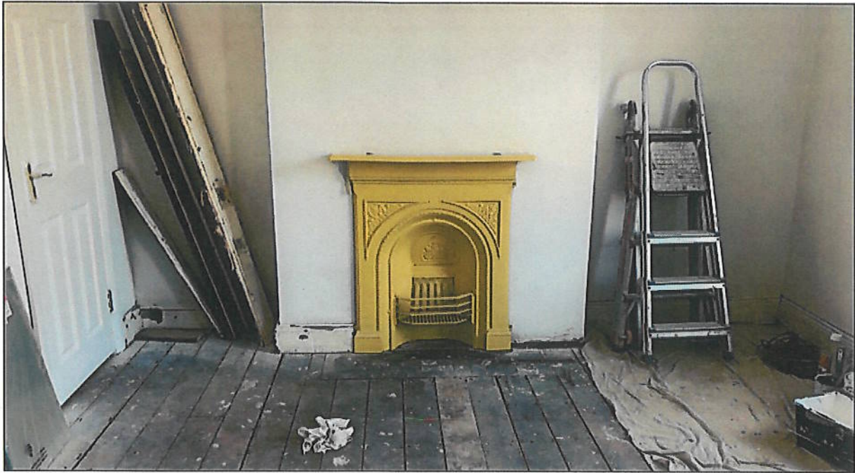
Insertion of traditional type fire places in lieu of inappropriate fireplaces previously existed
