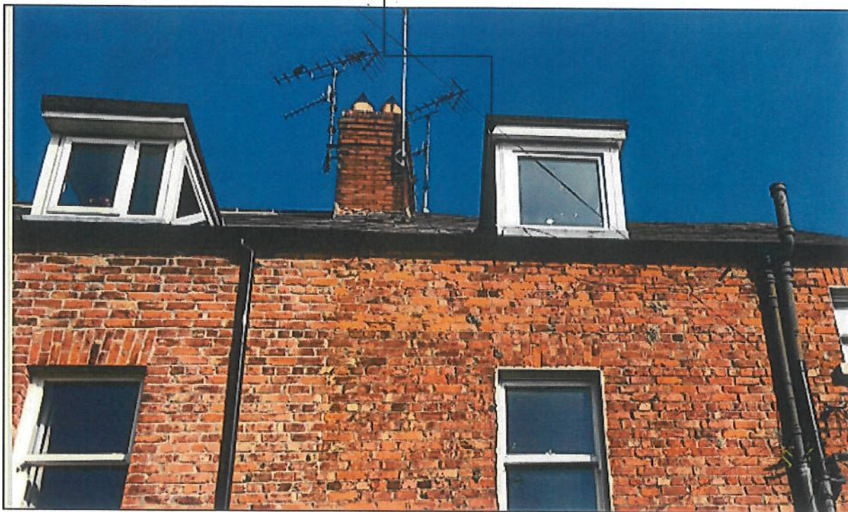
Attic window replaced with PVC window
