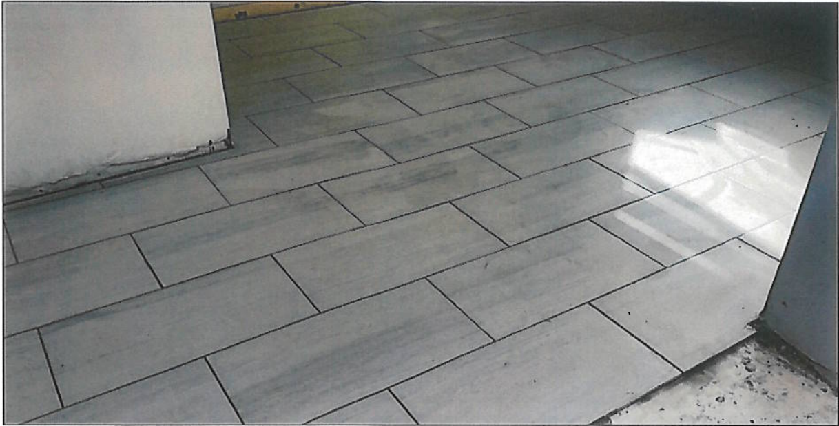
Internal tiling to rear extension to rear single storey (not thought to be part of original house that has been constructed which has been modernised in part (tiles laid on concrete surface) b=new skirting, plumbing & wiring also.
