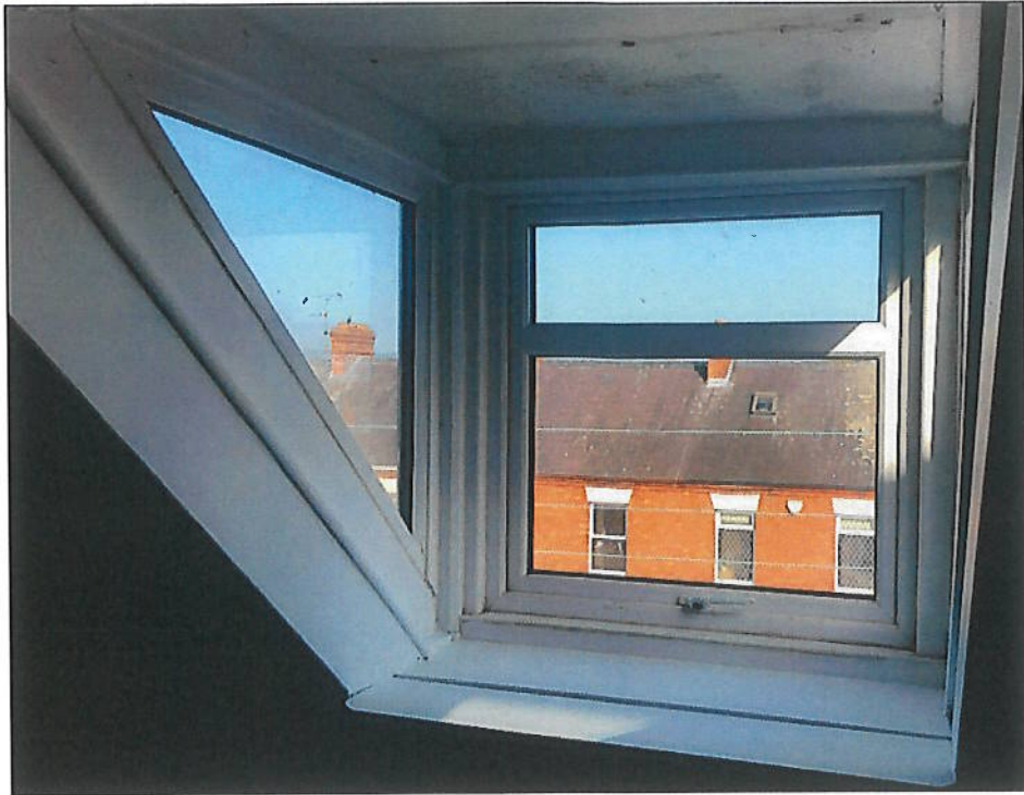
Works done to external window which has been replaced a former dilapidated wooden window
