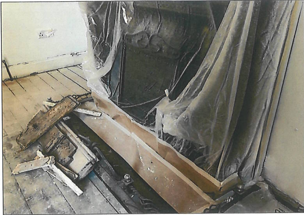
Figure 1 New fireplace to replace original which wasn't original
