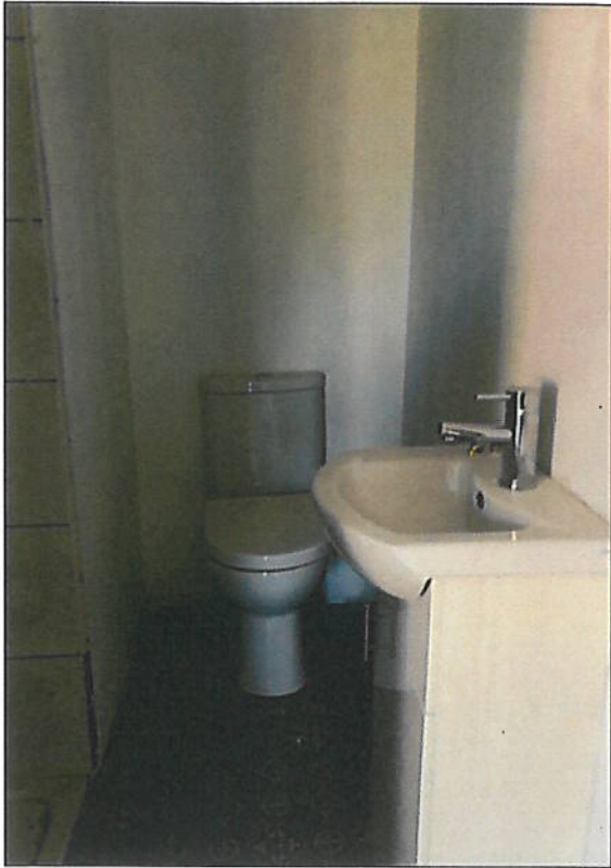
New toilet works
