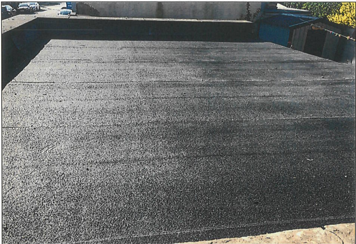
Works already carried out to existing flat roof extension where roof re-felted + resealed etc + new pipe-work inserted.
