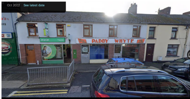
Above: subject building as of October 2022 (Google Streetview)
