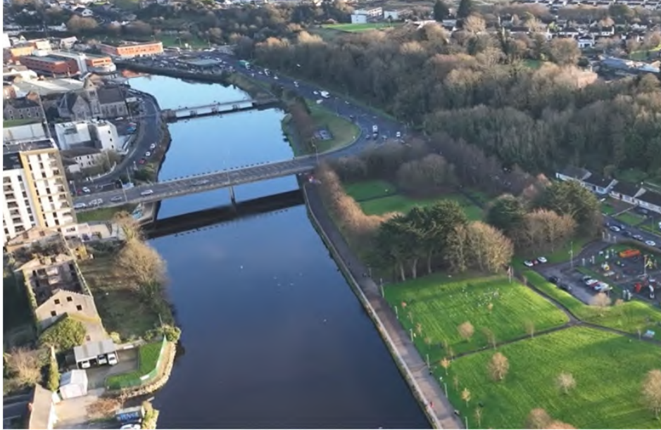
Plate 9. Aerial photograph taken at 120m elevation over the northern bank of the Boyne River facing in an easterly direction showing George’s Bridge and St. Dominic’s Bridge further downstream
