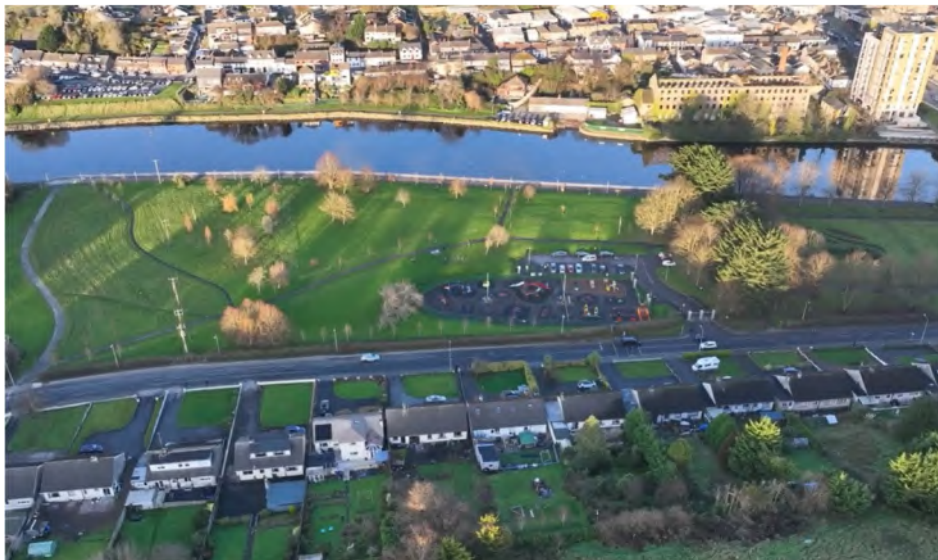
Plate 1. UAV Aerial photograph of site taken at 120m elevation to the south of the Rathmullan Road residential area to the south of the site facing in a northerly direction.
