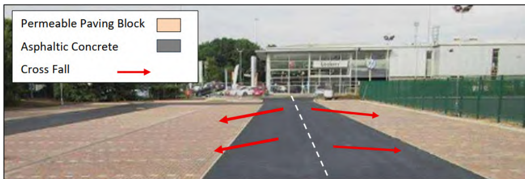
Plate 18. Proposed Surface Water Management showing asphalt sloped to adjacent permeable paving block (indicative only)
