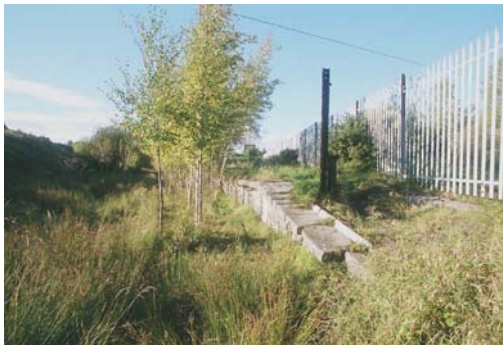
02101_02 FWH 04/10/2007 South end of Ardee side of Island Platform, from south.
