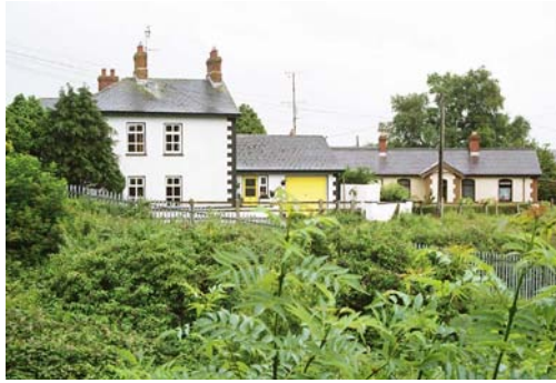
02101_05 FWH 09/07/2007 Station master's house (left) and cottages (right) from east.
