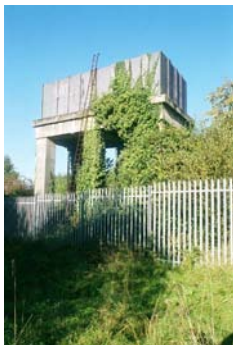
02101_04 FWH 04/10/2007 Water tank from west.
