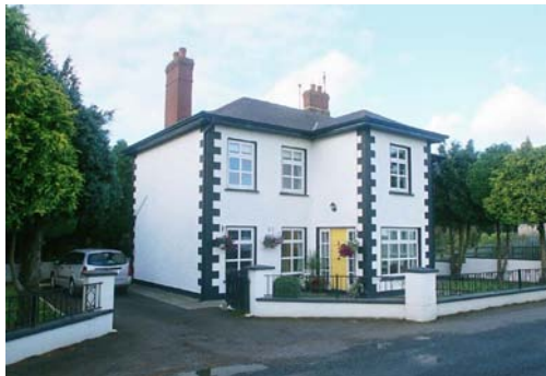
02101_07 FWH 04/10/2007 Station master's house from SW showing modern extensions.
