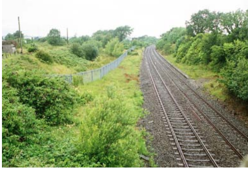
02101_01 FWH 09/07/2007 General view from south.
