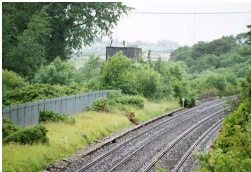
02101_03 FWH 09/07/2007 Water tower from SE.
