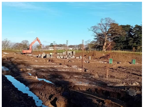
Column Steel reinforcement from foundations
