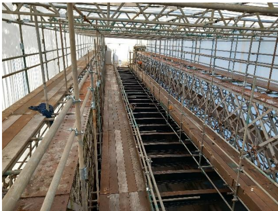
Obelisk Bridge inside view of encapsulation works
