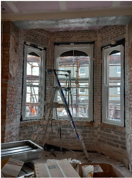
Block B Bay Windows installation
