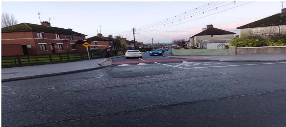
Low-Cost Safety Works at Priest Lane, Drogheda
