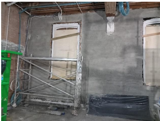
Block C Central Room scratch coat plaster coat application
