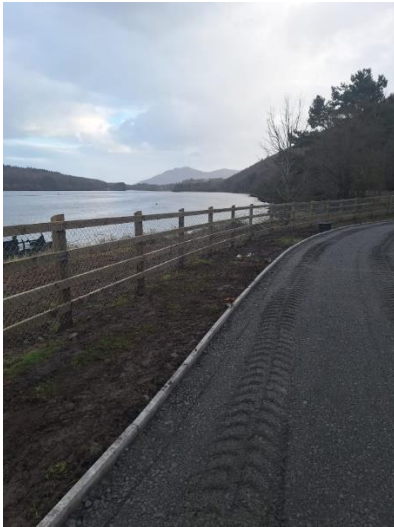
Works in Victoria Lock in NI
