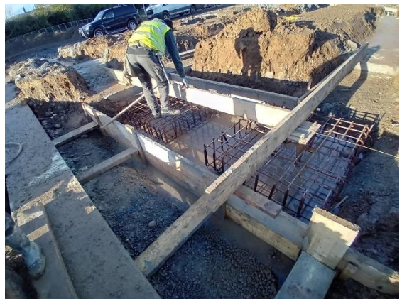
Foundations being prepared.
