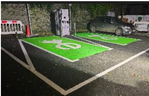
Works completed Ardee Car-park .
