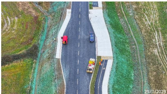
Road Marking Works in Progress at bus bays and cycle tracks
