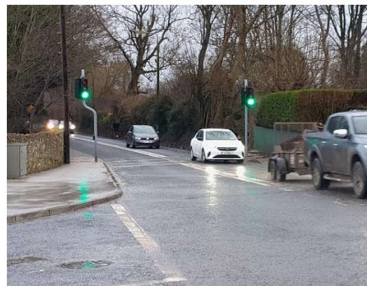
New pedestrian crossing At N53/Mt Avenue/ Mill Road
