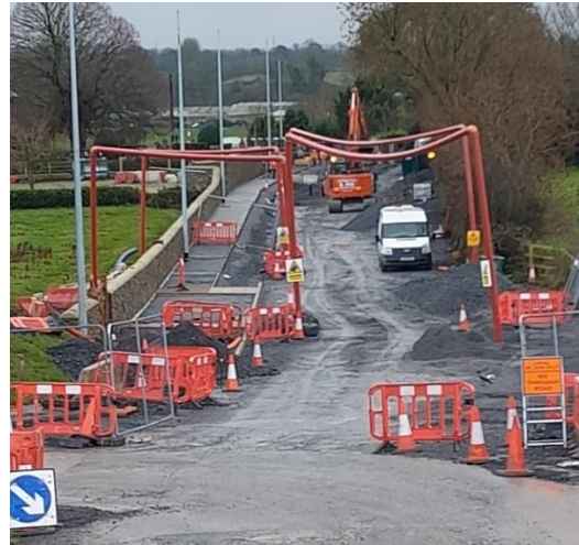
Footpath, public lighting, services and drainage south of Headford entrance.
