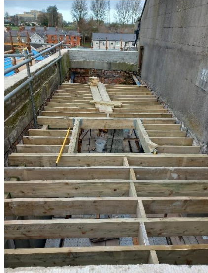
Block E Annex Building : Roof construction
