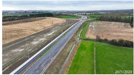
Public lighting and planting in progress looking west
