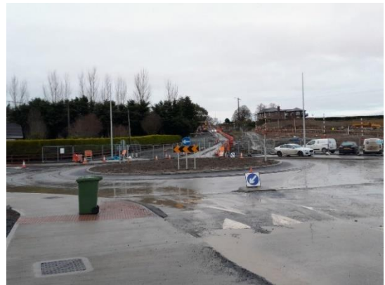
Roundabout entrance at council housing entrance
