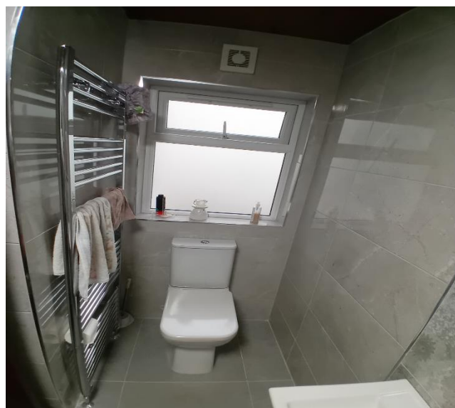
Bathroom Adaptation completed in Dundalk/Carlingford, part-funded with a Housing Grant for Disabled Persons
