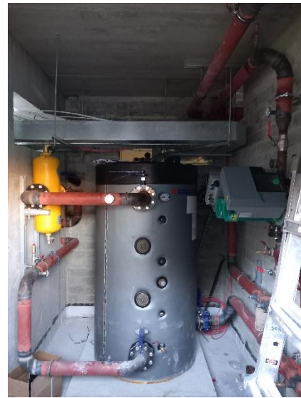
Block N: Hot Water Plant Room installation works
