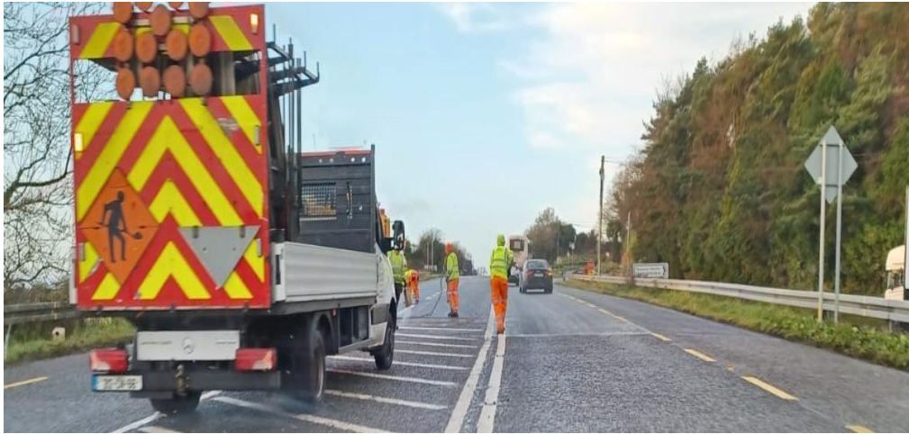
New road studs at Monasterboice
