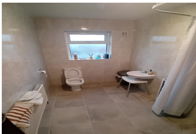
Bathroom Adaptation completed in December in Ardee, Part-funded with a Housing Grant for Disabled Persons
