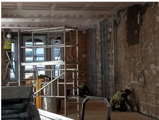
Block B Wall lining frame support system install
