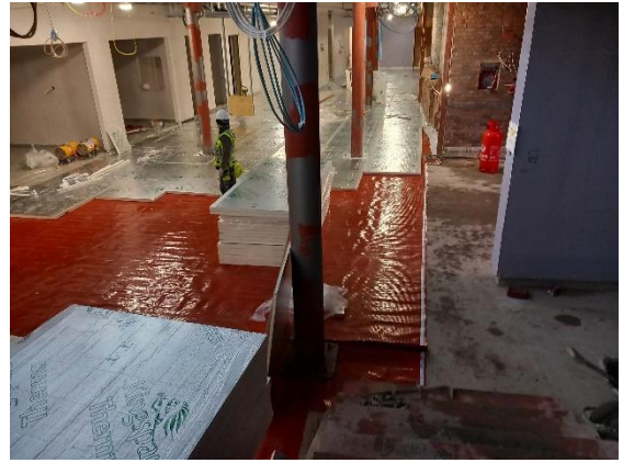
Block N Floor build up radon with insulation over.
