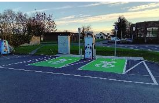
Works completed Dundalk (Tennis Club)
