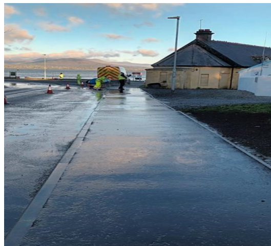
Footpath improvements at Greenore
