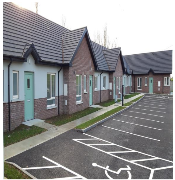
Turnkey Units in Park Green Coulter Place Dundalk
