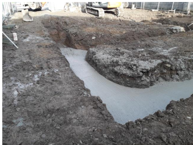
Foundations for new housing unit-Gort Uaine, Clogherhead
