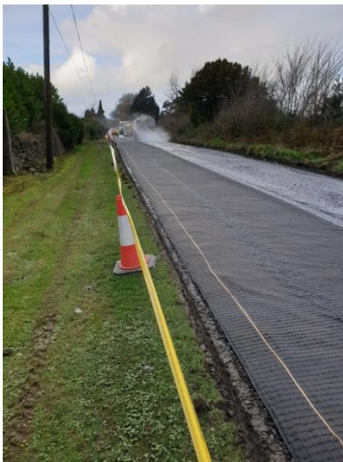
Road repairs in Gallstown
