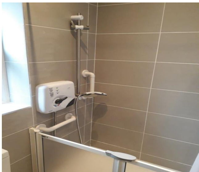
Housing Adaptation Grant, Level Access Shower
