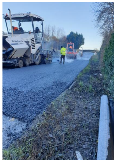
Road repairs on the N52
