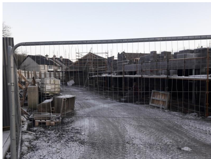
Construction progress new housing units – Doire Beag, Collon
