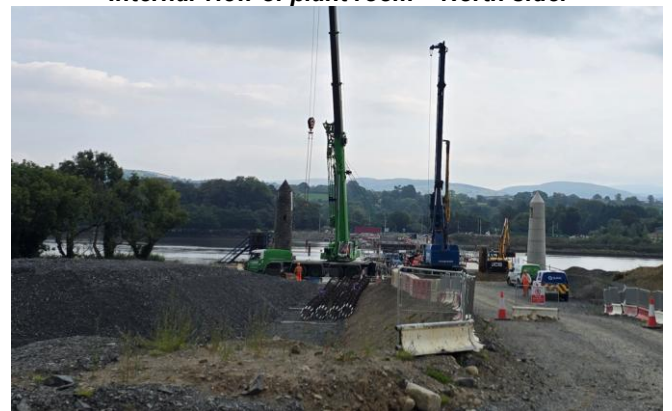
Piling for temporary support tower.
