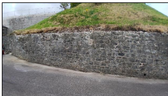
Wall Repairs at Millmount
