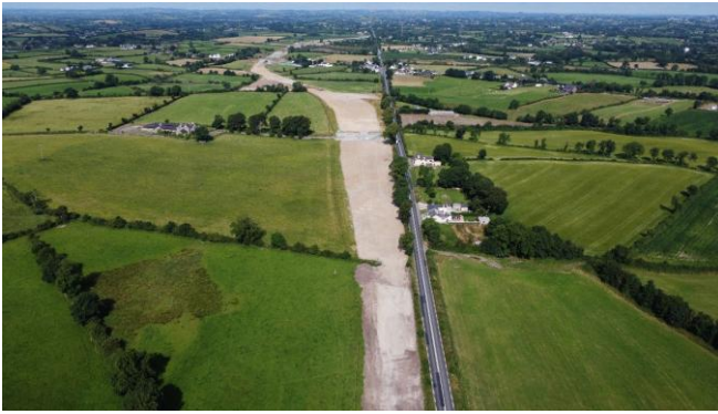
Drone image of overview of works on the N53
