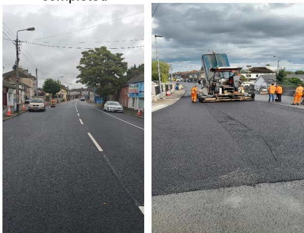
Hill Street Bridge + Anne Street Resurfacing
