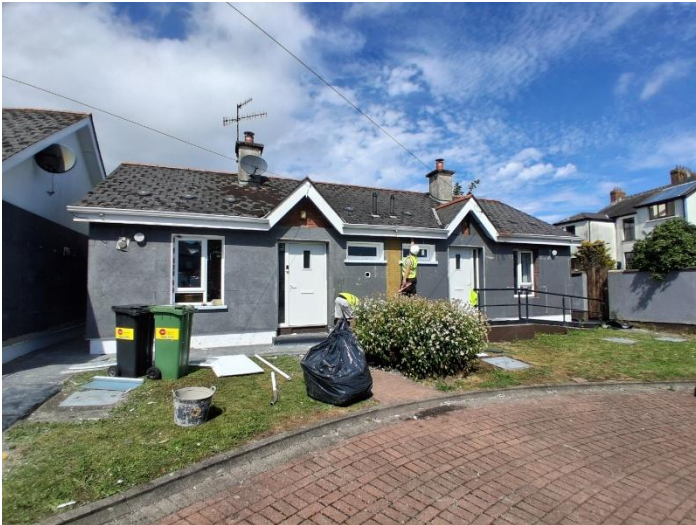
EWI Installation in Dundalk Street, Carlingford
