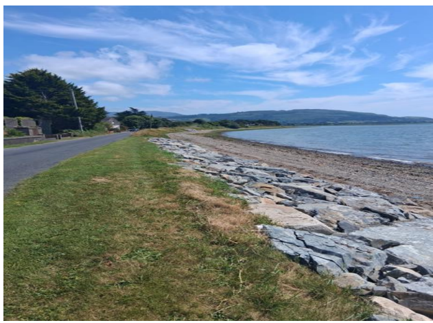
Coastal erosion protection works at Bellurgan
