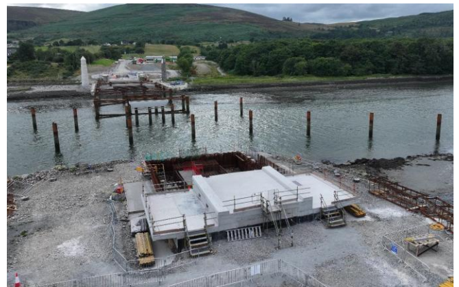
Northside – Overview of works at the Plant Room deck
