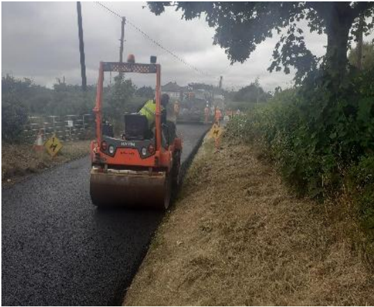
New Road Resurfacing at The Dales, Clogherhead
