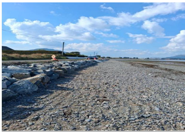
Coastal erosion protection works at Ballagan
