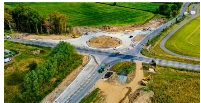
PANCR Phase 2- Roundabout Construction R166
