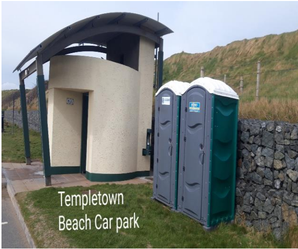
New Public Water Dispenser at Templetown Beach
