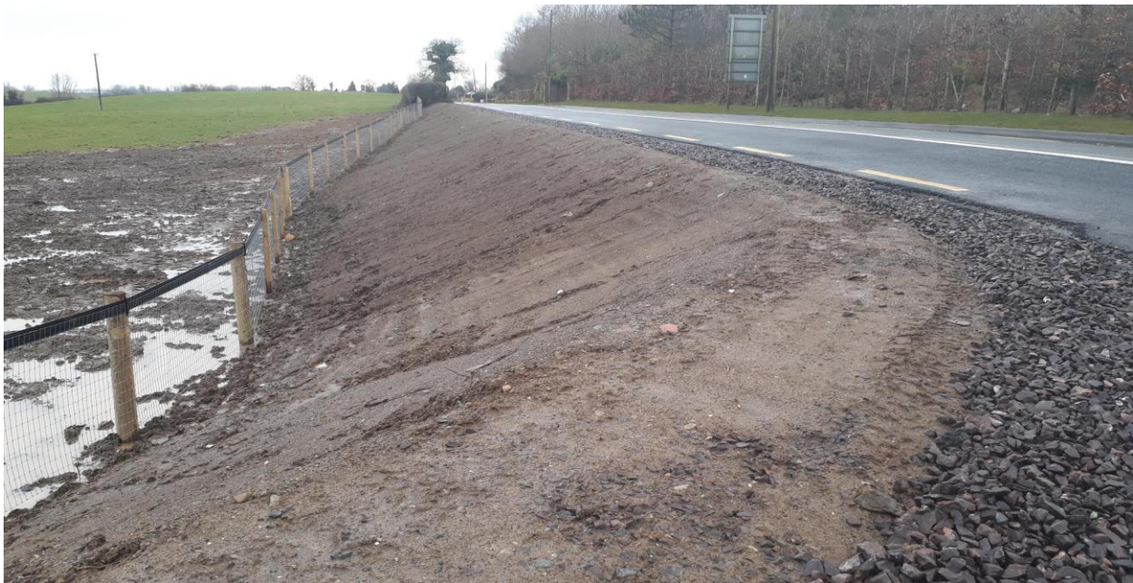
N52 Embankment at Ballygowan substantially completed
