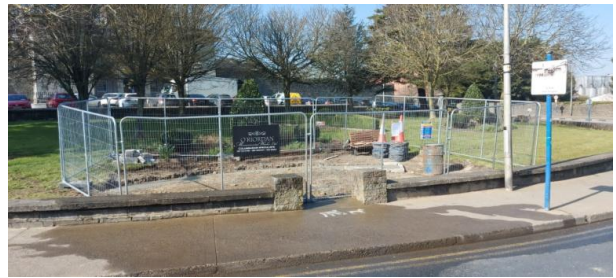
Commencement of the installation of the Dundalk War Memorial
