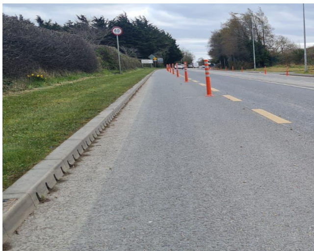
Cycle lanes on the North Road Drogheda
