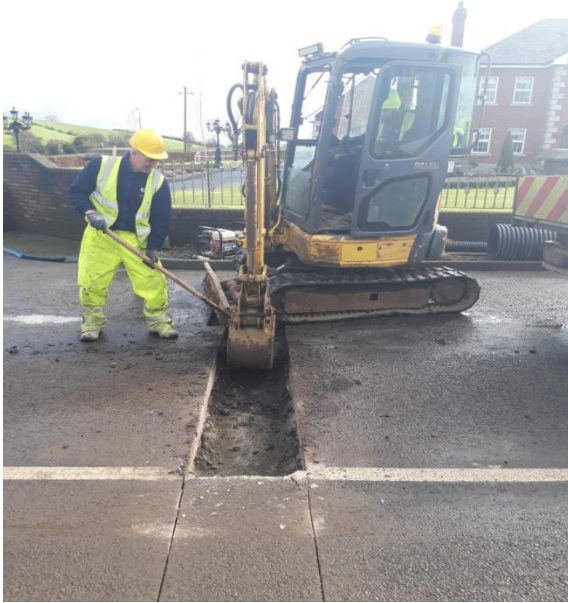
Drainage works at Drumbilla Sky Hill
