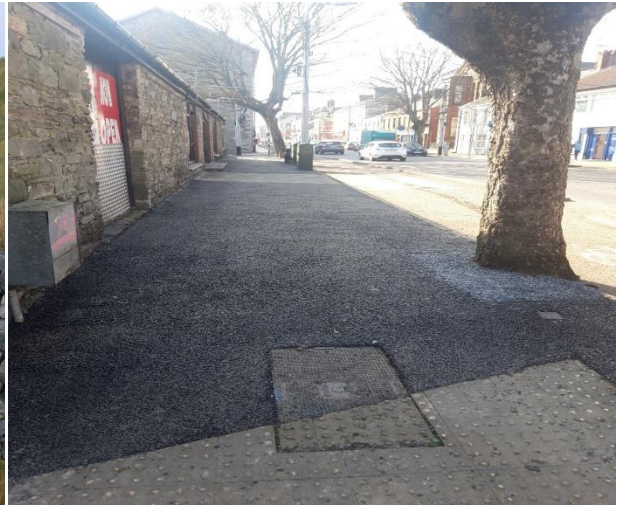
Footpath reinstatement at Jocelyn Street
