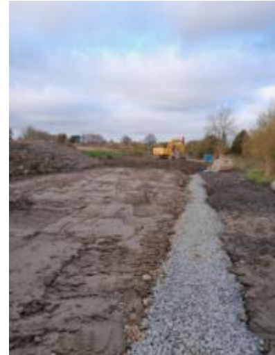
Backfilling of Pipeline
