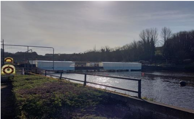
St. Dominick's Bridge- Bridge Encapsulation
