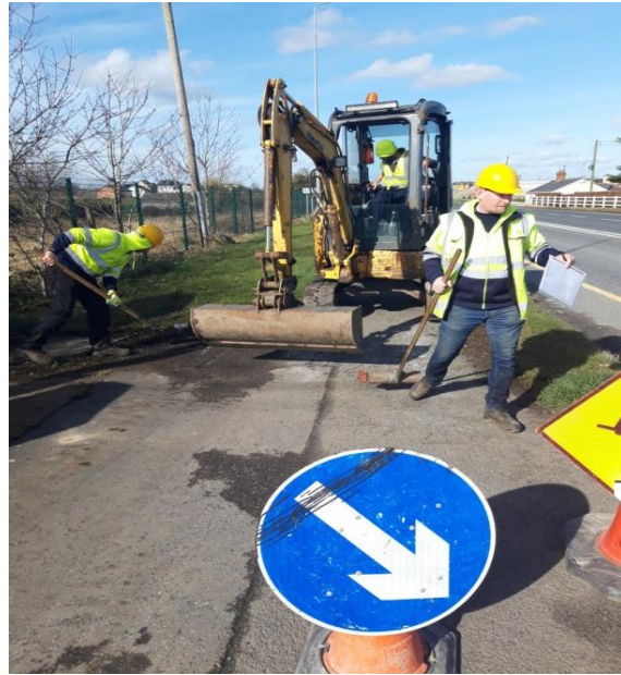
Footpath maintenance/clearing at Greengates
