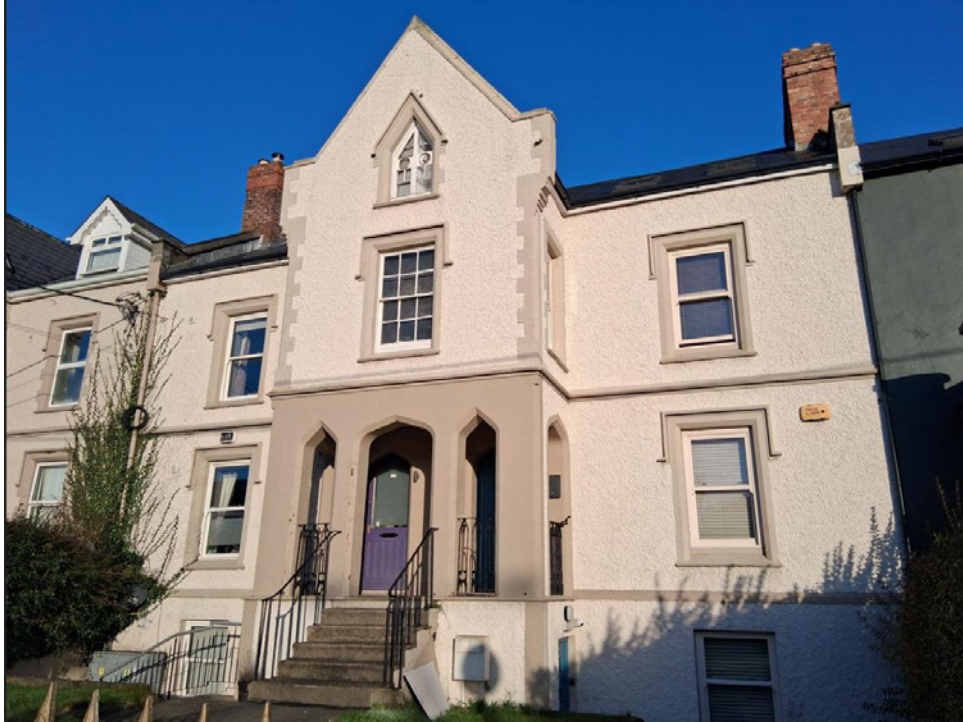
Figure 2: Existing dwelling (taken 16/12/2025.)
