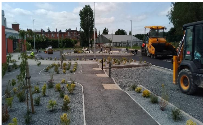
Bitmac works to Access Road 20th July 2026
