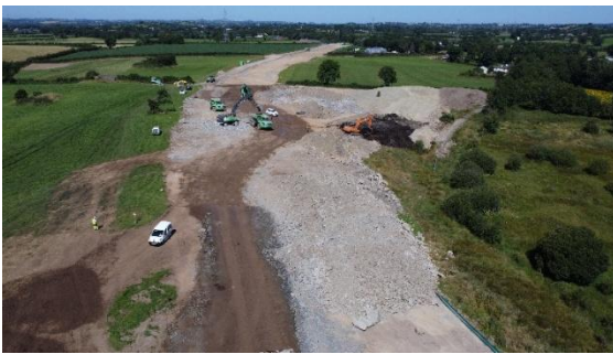
Construction Works of realigned N53 overview
