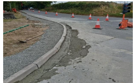
Newly laid kerb line
