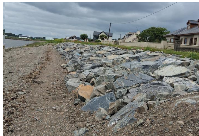
Coastal Protection Measures Bellurgan
