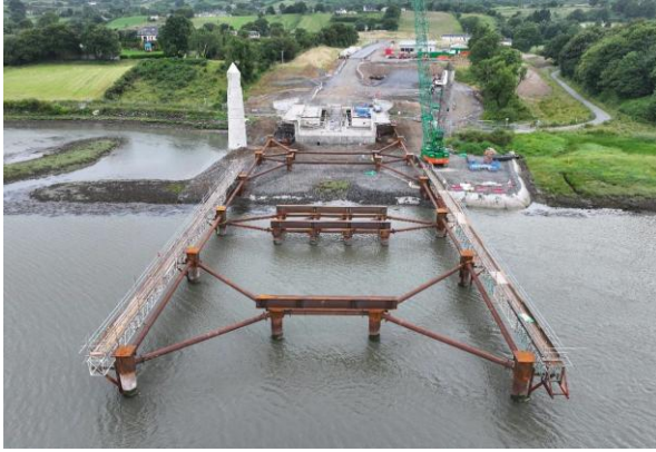
Temporary skid beam bracing installed.
