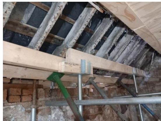
Structural bracing to roof
