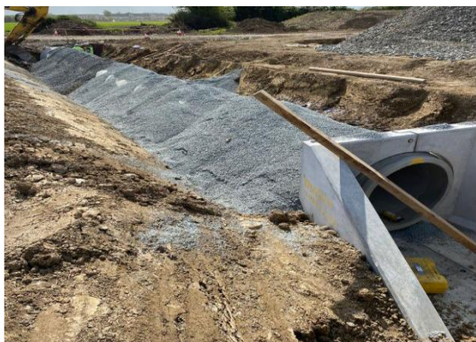
CH300 – 1200mm Culvert
