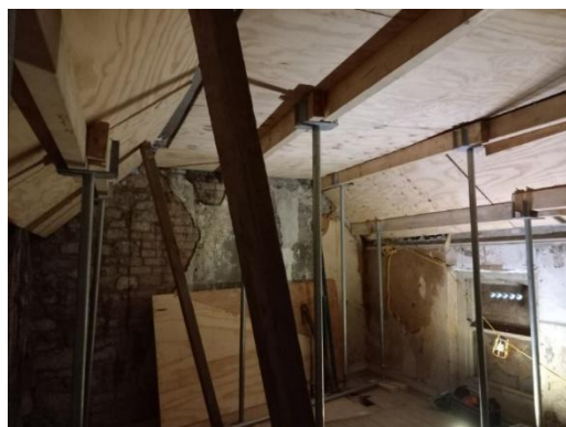
Roof Safeguarding Works
