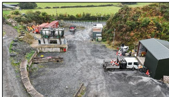
The existing Bush Depot at Ballaverty
