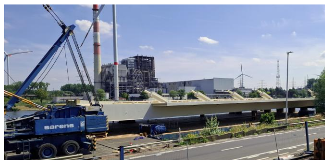
Fixed Deck 1 moored at Sarens Yard
