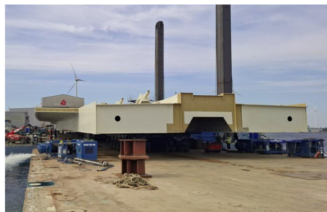
Load out of Fixed Deck 1 onto Barge
