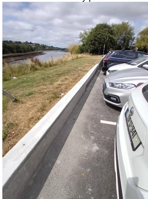
Mell Road Carpark boundary wall
