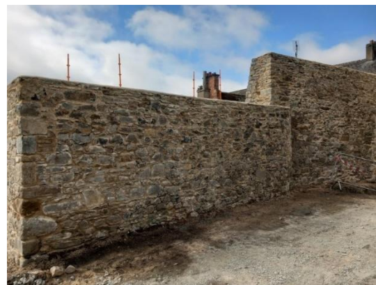
Completion of Rubble Stone Walls
