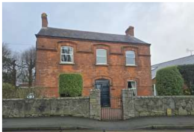
Above: Front of protected structure
