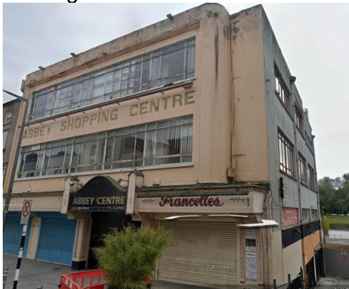
Fig 1: Google image of the subject building.
