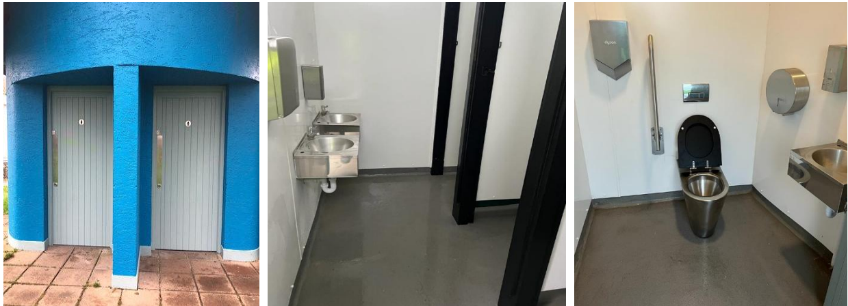
Completed work in Carlingford and Gyles Quay Public Toilets
