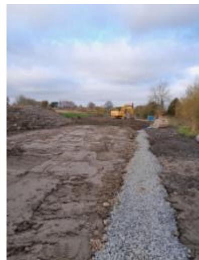
Backfilling of Pipeline
