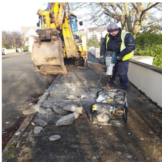
Footpath repairs in the Ferns Blackrock
