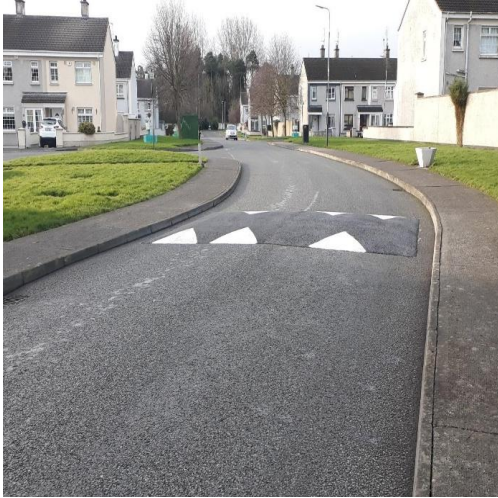
New Speed ramp installed in Ferdia Park
