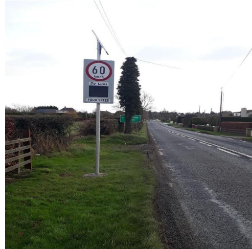
New flashing Speed Warning Sign Installed on Ardee N52 Kells Road approach to Ardee
