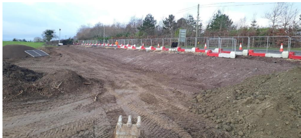
N52 Ardee to Kells road Embankment Strengthening Works at Ballygowan
