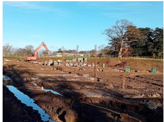
Column Steel reinforcement from foundations
