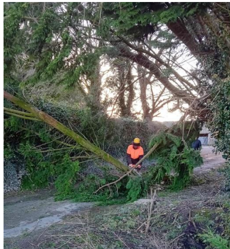
LCC removing fallen tree on L-3167 Rathiddy Road Knockbridge
