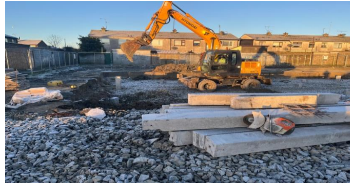
Muirhevnamore Infill Site, Dundalk – 11 housing units construction in progress
