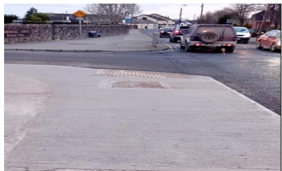
R170 Hale Street, Ardee after works.
