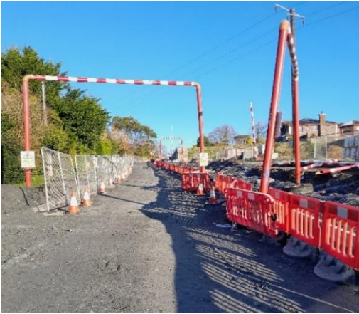
Kerbing and services along Council Housing frontage.
