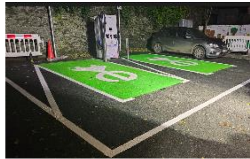
Works completed Ardee Car-park .
