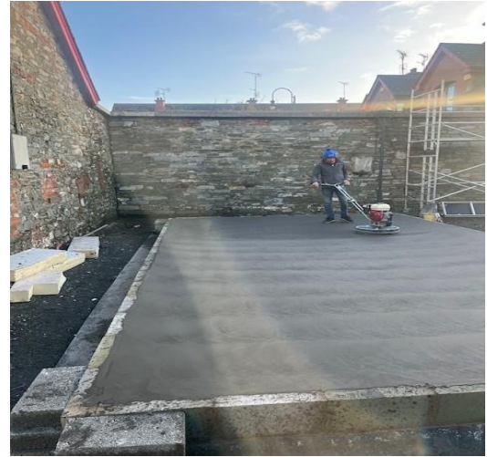
Constructing the Floor for the Learning Pod
