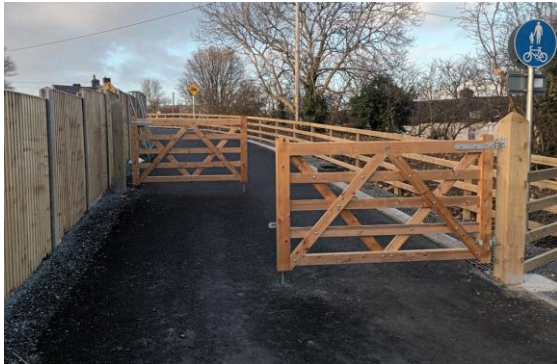
Greenway access control points installed at culvert
