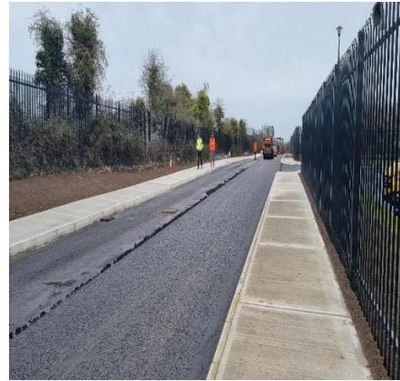
New carriageway with footpaths
