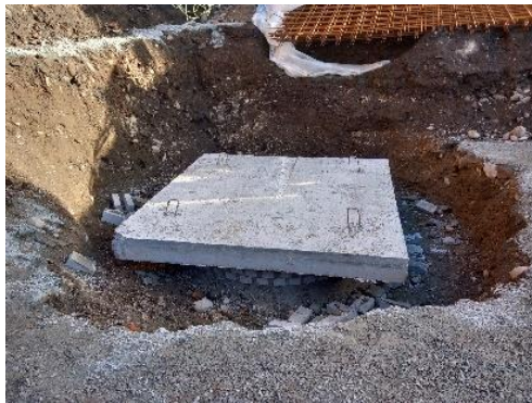
Block C Well Capping
