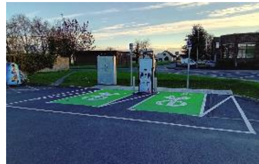
Works completed Dundalk (Tennis Club)
