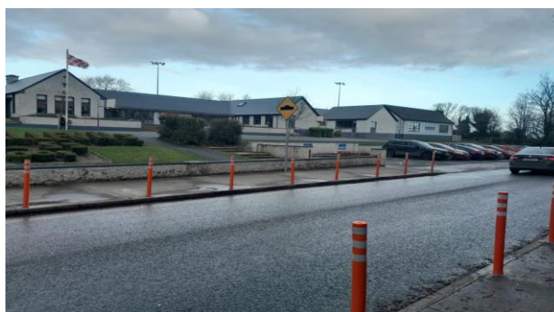
New Bollards installed at Tullyallen School on the LP-2318-17
