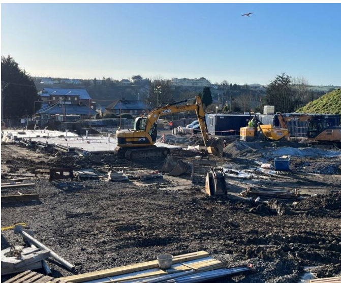
Boice Court, Drogheda - 72 housing units construction in progress
