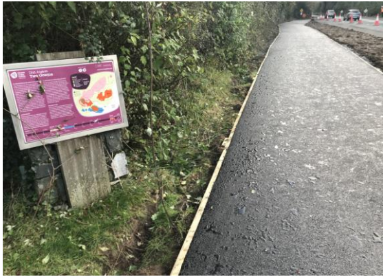
Works in Section 1 Carlingford
