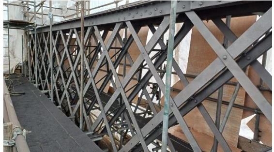
Obelisk Bridge Section of shotblasted steel
