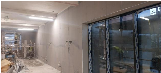
Block B Council Chamber Exhibition space fit out
