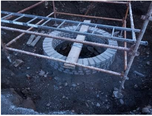
Block C Well Capping
