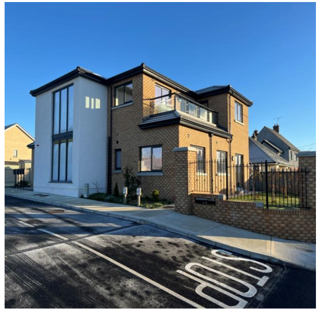
Mount Avenue, Dundalk – construction of 93 housing units in progress.
