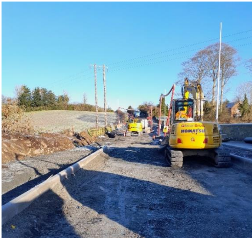
Kerbing, ESB ducting, drainage and service provision approaching Headford
