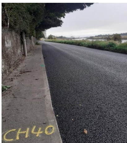
Road Works Programme, Drogheda
