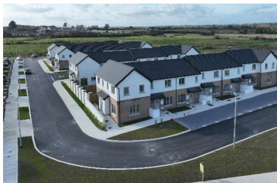
Ferrard Park, Drogheda – Turnkey Scheme
