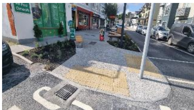
New Paving & Planting – Omeath Placemaking Scheme
