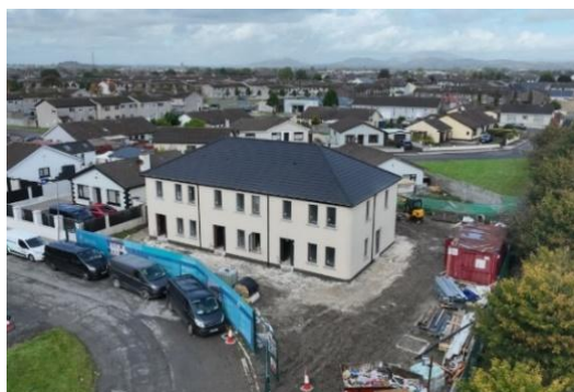
Grange Close, Dundalk – Pilot 3D Construction Printed Scheme
