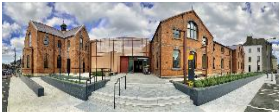
View of Refurbished Civic Offices, Drogheda
