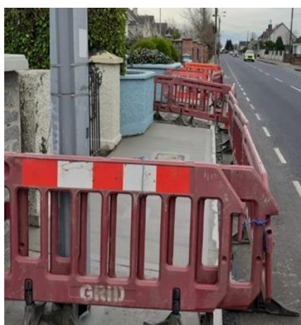
Footpath works – Avenue Road
