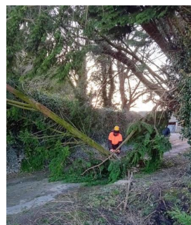
LCC staff removing storm tree
