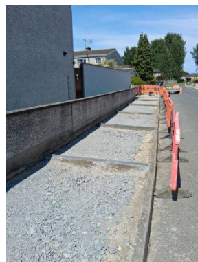
Footpath improvement works.
