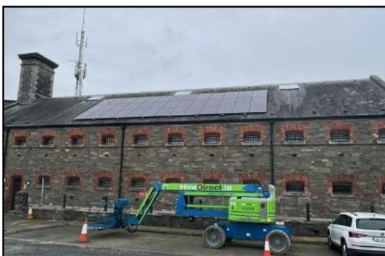
Installing Solar PV at the County Archives Building Dundalk
