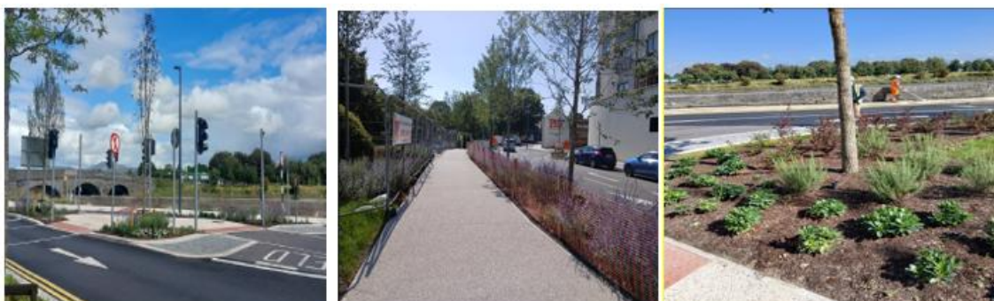
St Nicholas Quarter Phase 1 Public Realm Works
