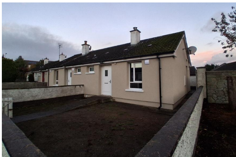
Mayfield Drive, Dundalk (example of Energy Efficiency Retrofit Programme)
