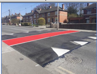
Traffic calming in Drogheda 2025 integrating pedestrian safety
