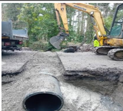
Drainage works and new culvert installed in Cooley
