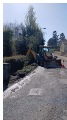
Drainage and Verge works
