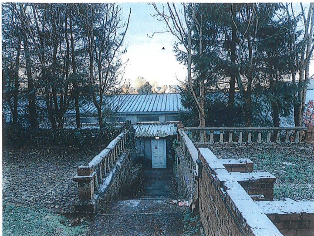
Figure 3: Views of existing swimming pool building roof.
