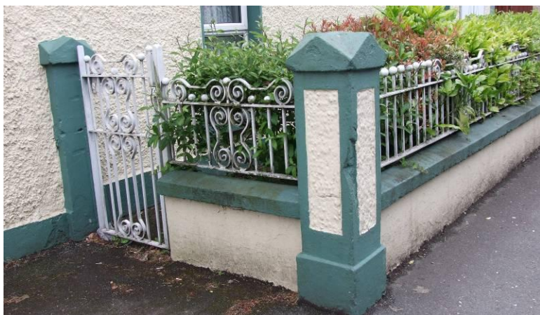
Fig. 129: Decorative ironwork on Dundalk Road
