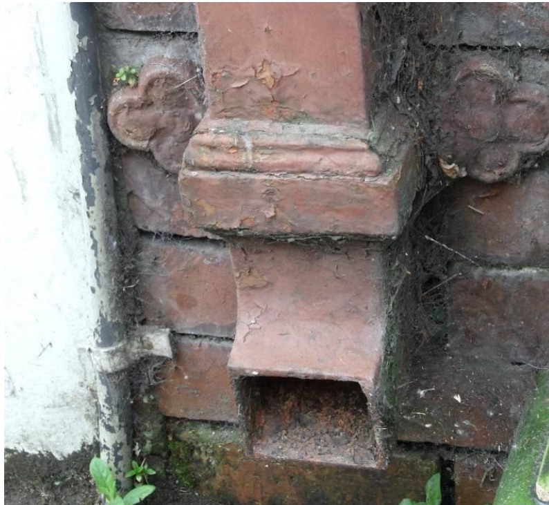
Fig. 108: Down pipe with decorative fixings, Bridge Street
