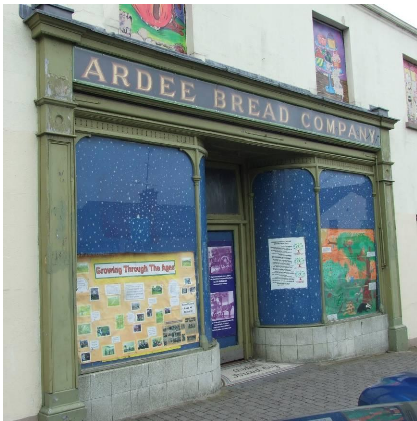
Fig. 123: Elaborate shopfront on Castle Street
