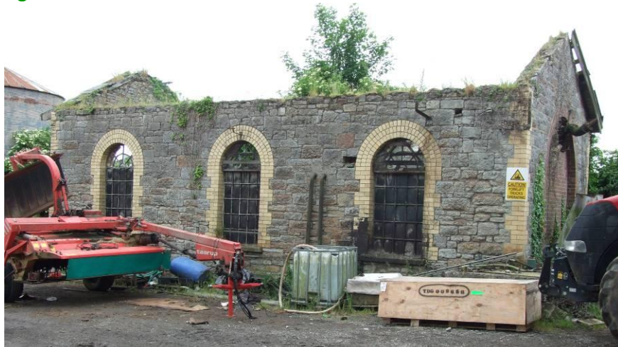
Fig. 67: Former Station Good Shed
