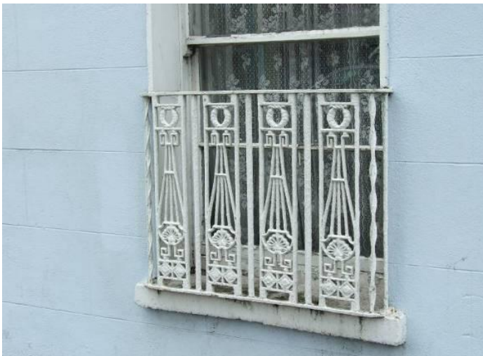
Fig. 120: Ironwork window guard on Castle Street
