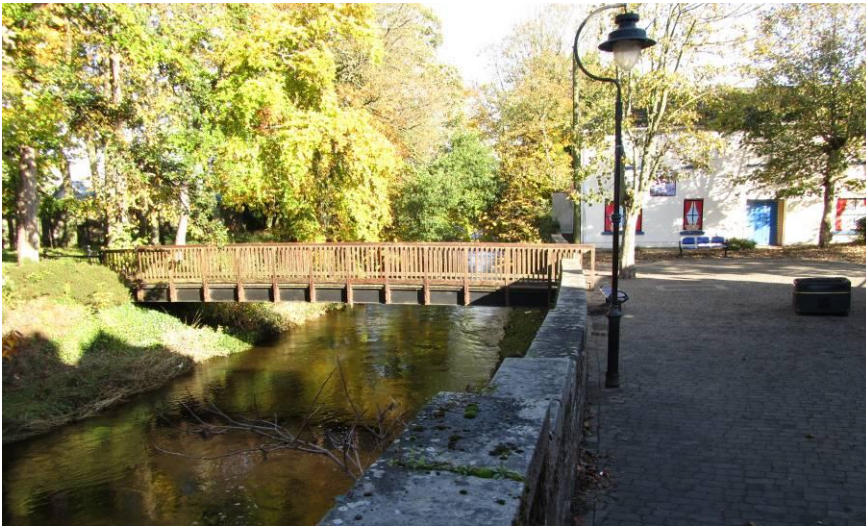
Fig. 83: Stone riverside wall and view east to park on former island
