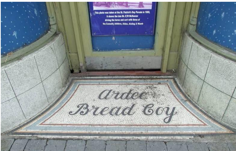
Fig. 101: Tiling to shop entrance on Castle Street
