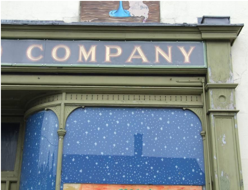
Fig. 25: Detail of shopfront on Castle Street
