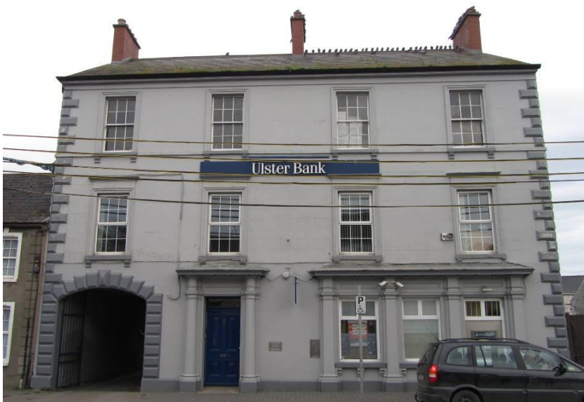
Fig. 39: Ulster Bank building
