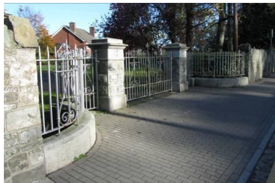
Fig. 97: right: cast iron gates and stone piers
