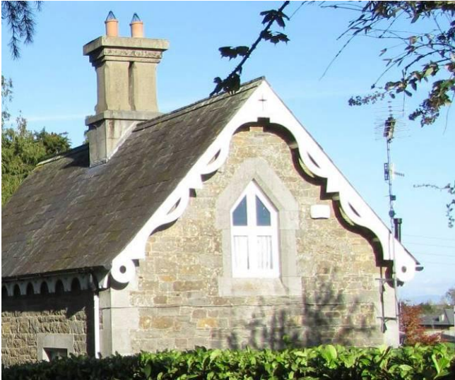
Fig. 107: Decorative bargeboards to convent gate lodge
