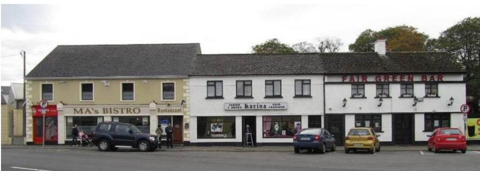
Fig. 35: Buildings south of the Fair Green intersection
