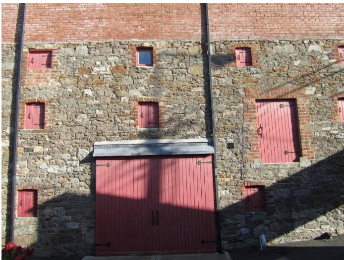
Fig. 112: Exposed brick and rubble stone wall
