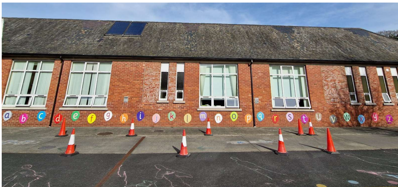
Figure 2: Image of roof where 34 no. solar panels to be erected.
