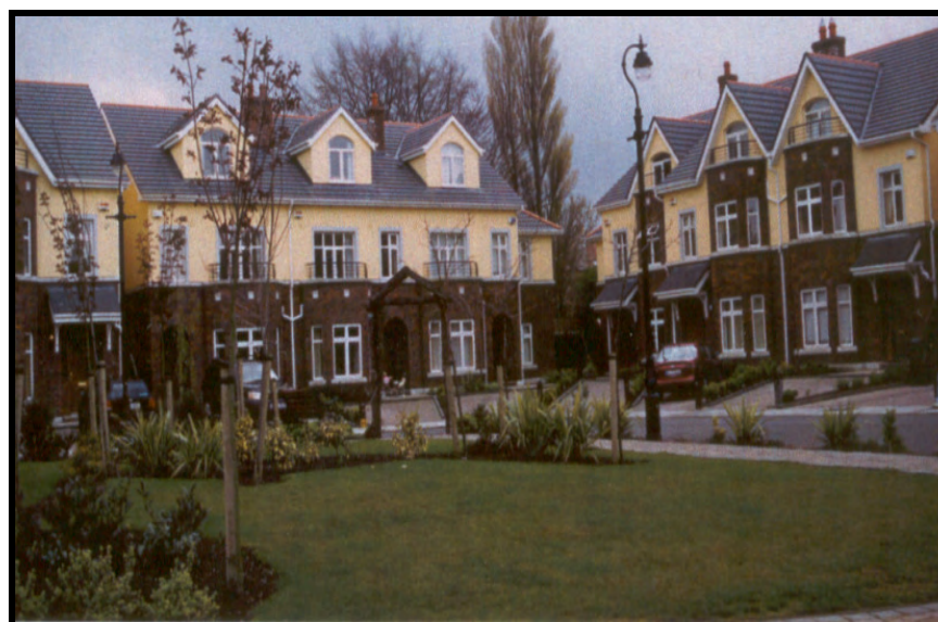
Plate 4.2 Housing overlooking open space
