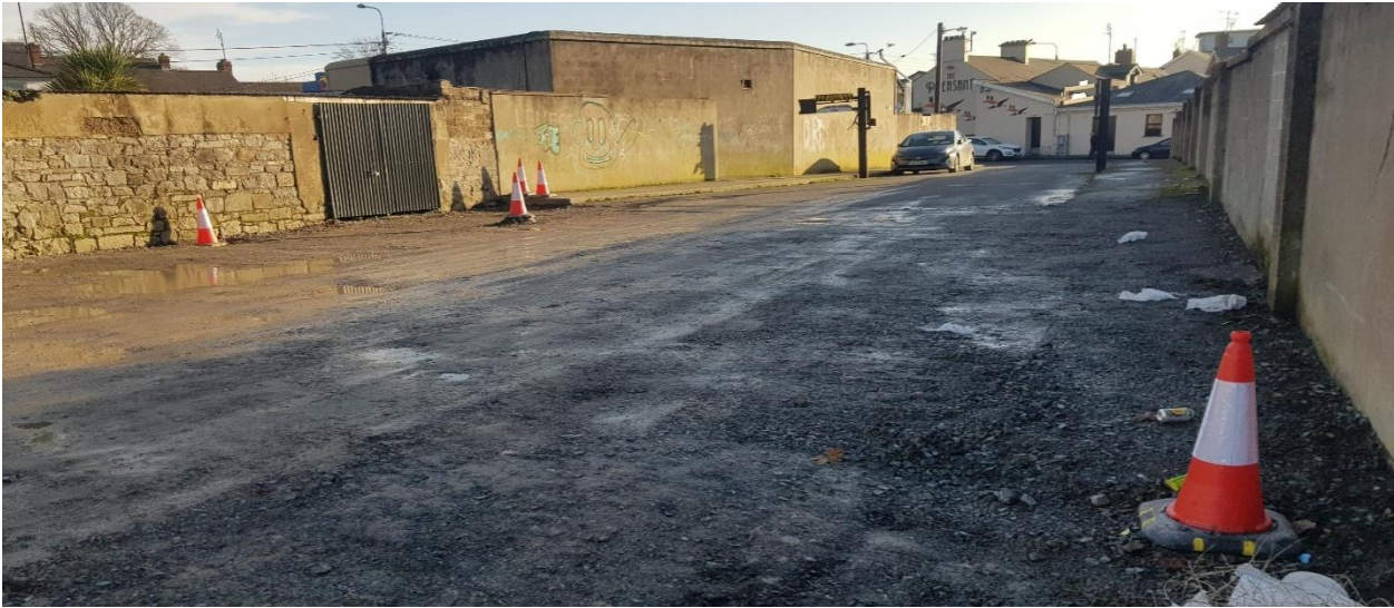
Sarah Gibney's Lane Drogheda Drainage work in progress
