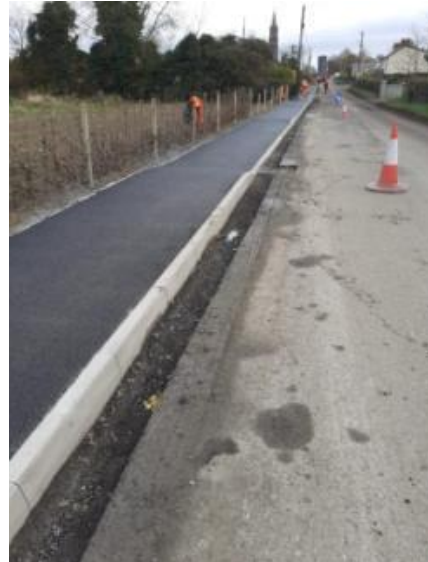
Stabannon Footpath- Works in Progress
