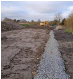
Backfilling of Pipeline
