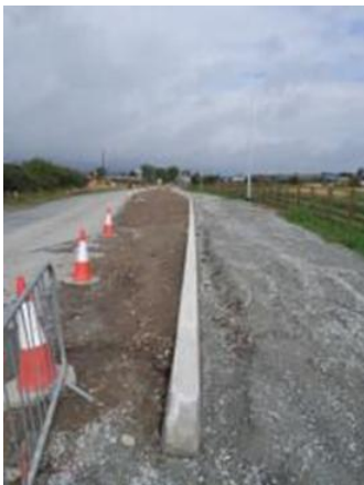
Footpath & Cycle lane Construction progress
