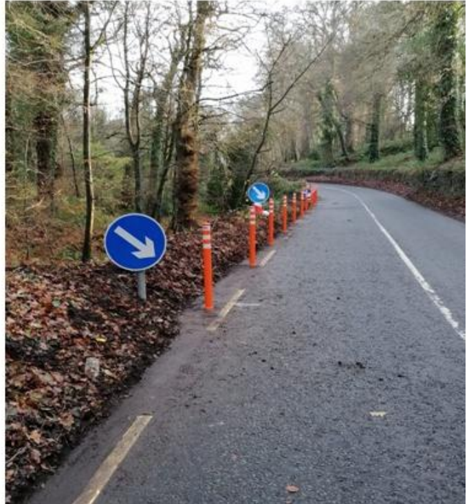
King William's Glen edge warning bollards LP-2321-0
