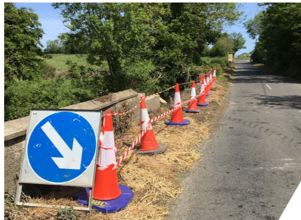
Bridge Damaged Togher Road.
