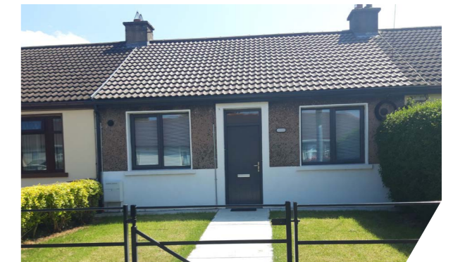
26 Culhane Street, Dundalk, acquired by Compulsory Purchase Order.
