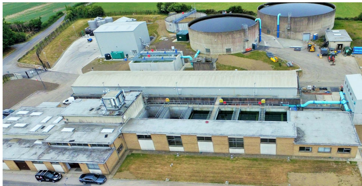
Staleen Water Treatment Plant.
