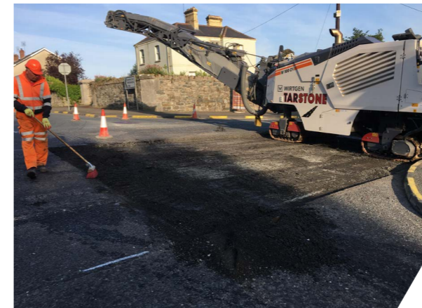
N2 Collon road works 1.
