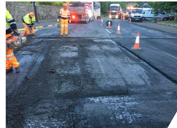
N2 Collon road works 2.
