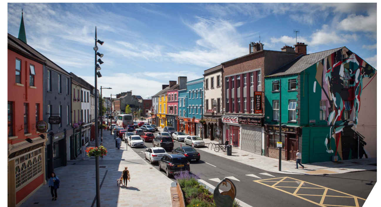
Church Street following the works on the Clanbrassil Street and St Nicholas' Quarter Rejuvenation Scheme.
