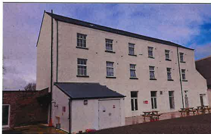
After works – Washroom removed + Fire-scape removed, alterations to opes
