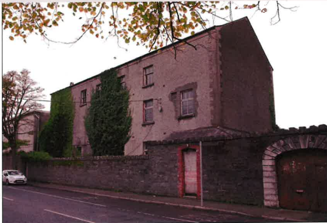
Castle Street Elevation pre works
