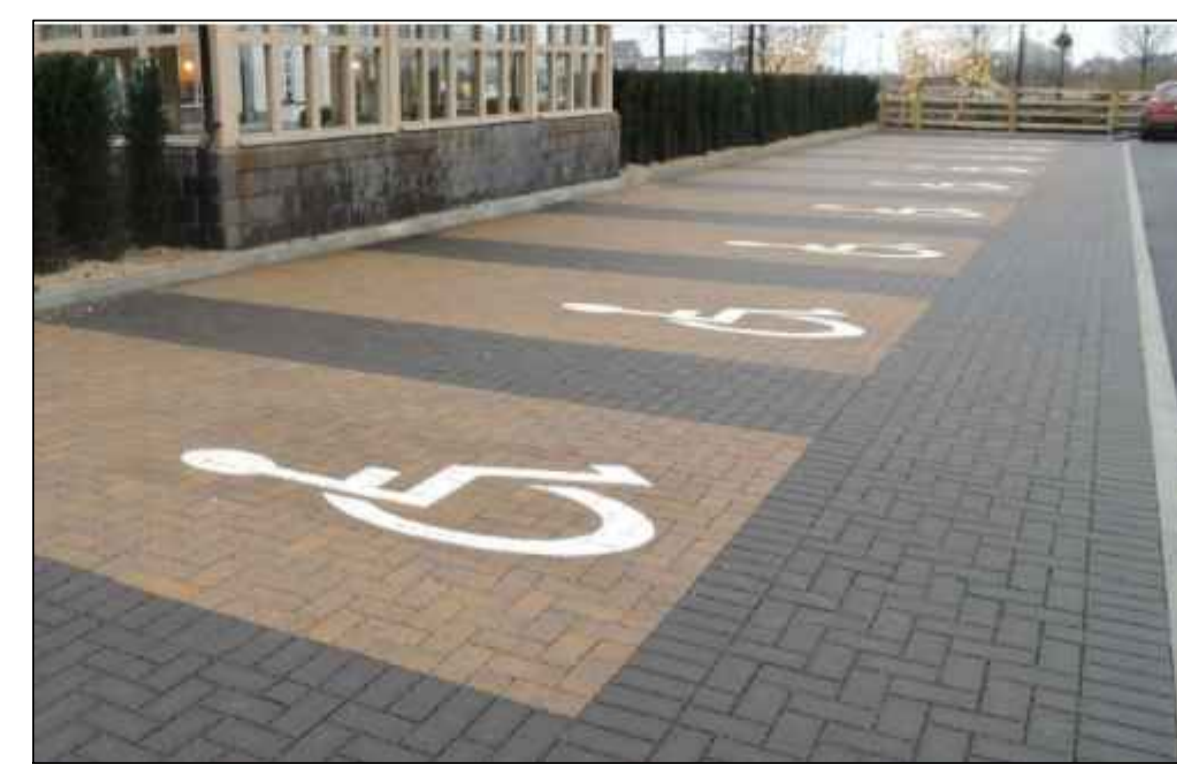
Typical Example of Permeable Paving
