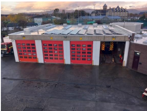
Figure:1.9 Solar Installation on Fire Station
