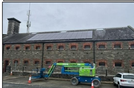
Photos: Installing Solar PV at the County Archives Building Dundalk
