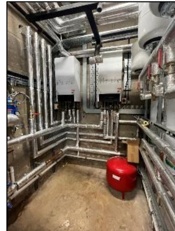
Photo: Enabling Works at Dundalk Fire Station for Energy Upgrade
