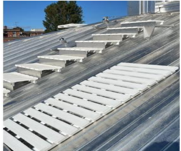
Roof Access completed
