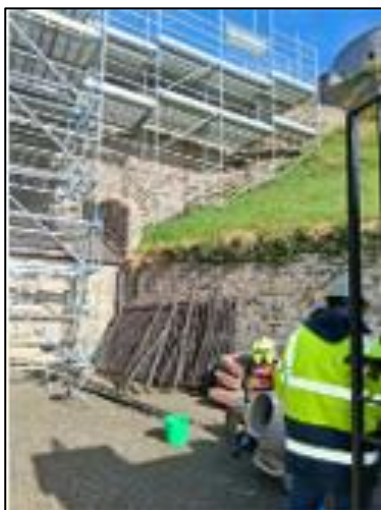
Photo: Wall Repairs at Millmount Drogheda & Temporary
