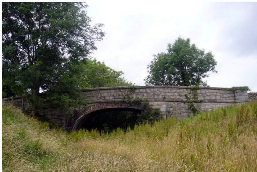
Plate 10.13 Former railway bridge on Greenore – Newry railway line. Note depth of cutting.
