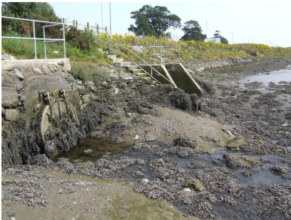
Plate 7.2.11 On the Down side, the shoreline is already artificially banked.
