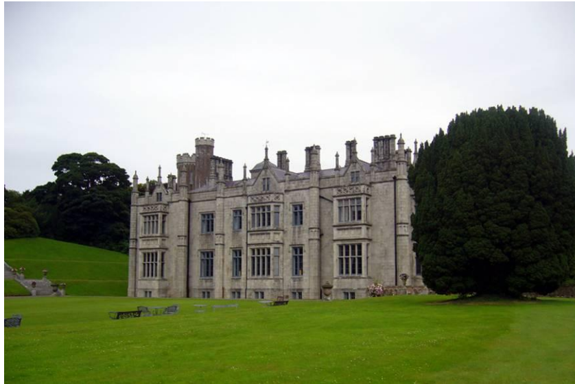
Plate 10.26 The Historic Building, Narrow Water House (HB 16/11/019)
