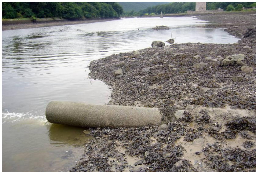
Plate 10.23 Sewage outfall pipe running across 'The Gut' to the Newry River.
