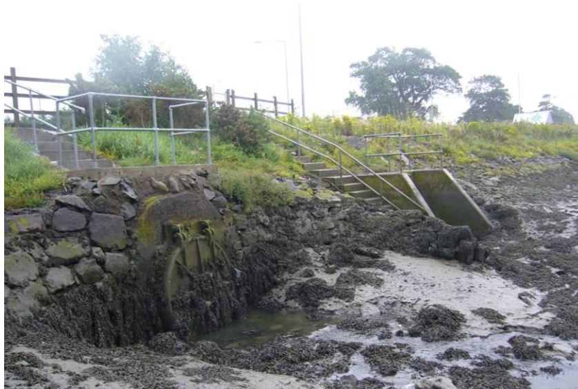
Plate 10.22 Embankment of roundabout on A2 Newry to Warrenpoint Road.
