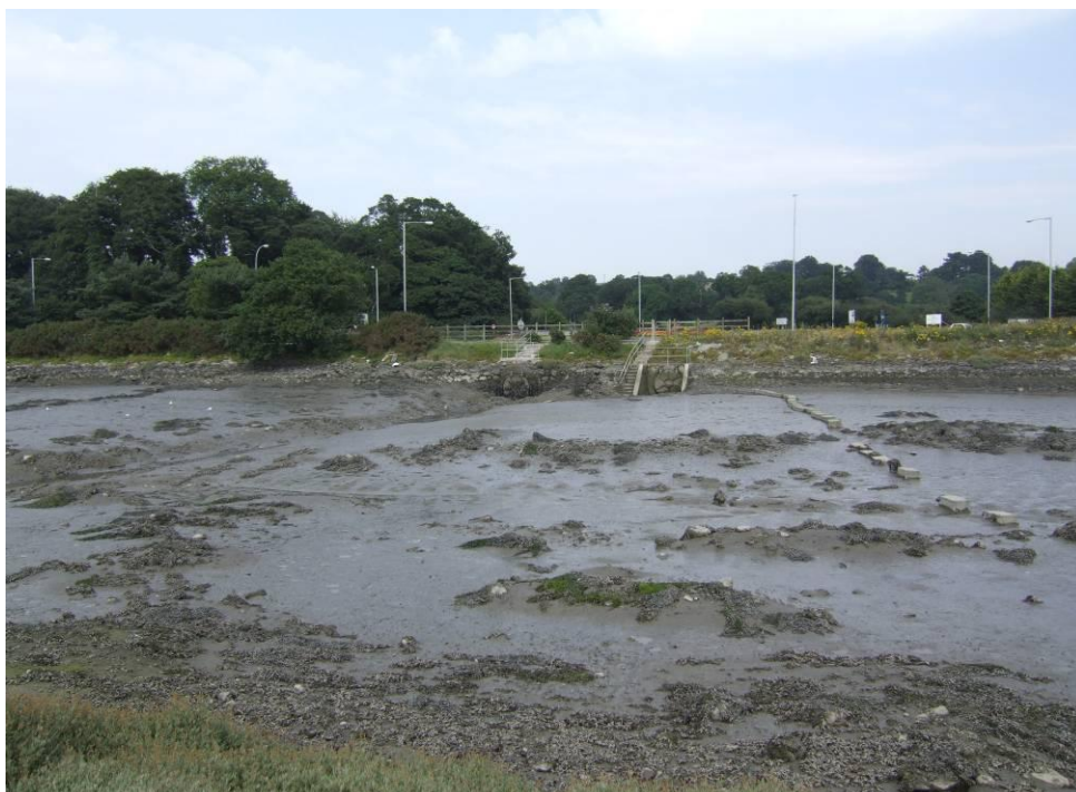
Plate 7.2.12 This area of mudflat will become very sheltered due to the presence of the proposed embankment, potentially resulting in the development of salt marsh vegetation. Looking north-east towards the A2.
