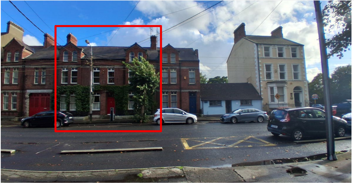
Fig 2: Existing Building taken from Jocelyn Street
