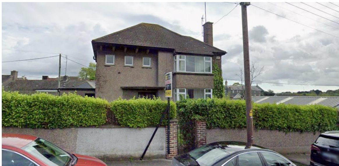
Front elevation from King St.
