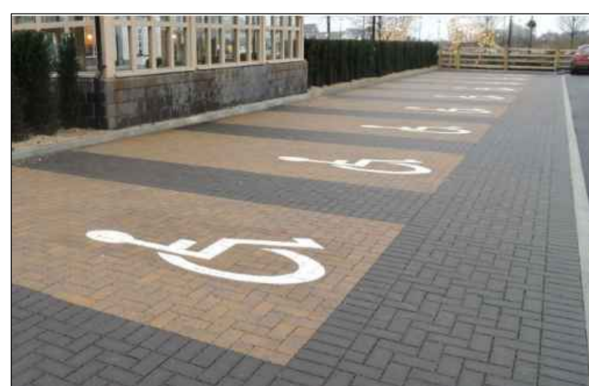
Typical Example of Permeable Paving
