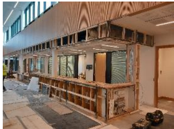
Customer Services Motor Tax Fit out
