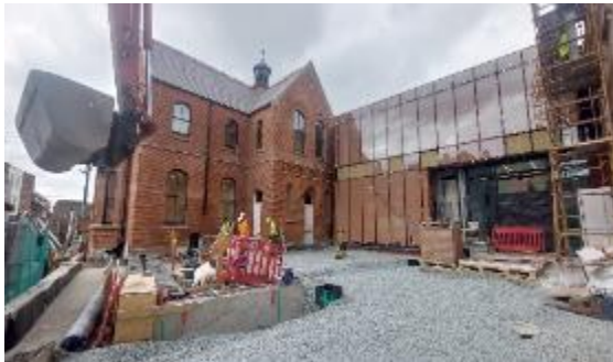
Block B and N (Main entrance) and ongoing external works.
