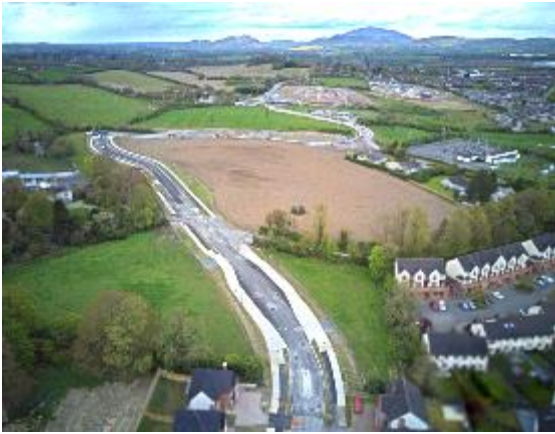
Aerial Photo of the full extent of the scheme.
