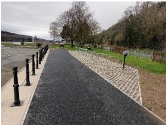
Works Complete in Victoria Lock in NI
