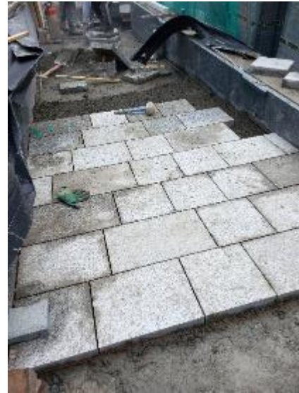
Paving to Ramp at Block B Council Chamber
