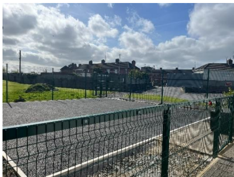
Capital works continuing at Lourdes Stadium
