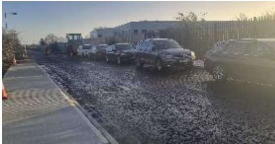
New carriageway with footpaths
