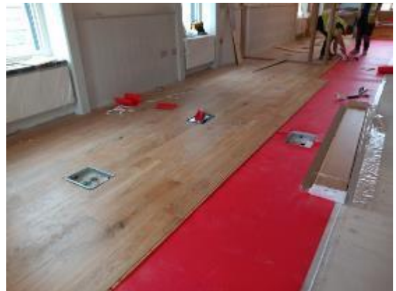
Block B Hardwood finished flooring
