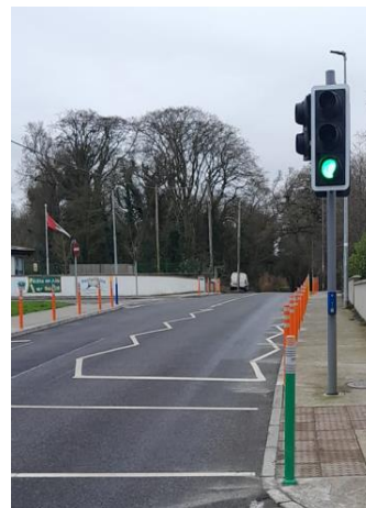
Bollards to Termonfeckin School R167
