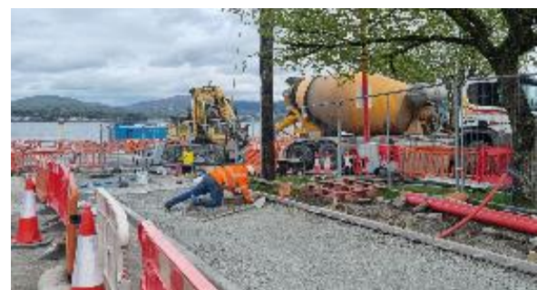
Preparation for installation of footpaths
