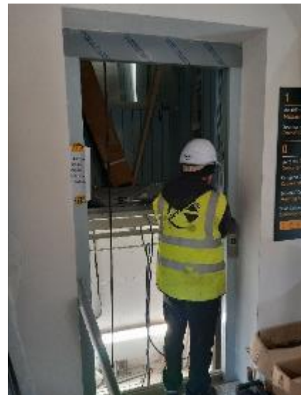
Block C Lift Testing and commissioning.
