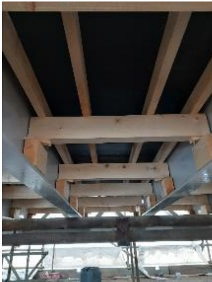
Shuttering to underside of Bridge Deck
