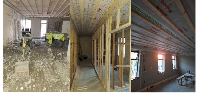
Construction Works Progressing at Former Bank for relocation of Dunleer Library
