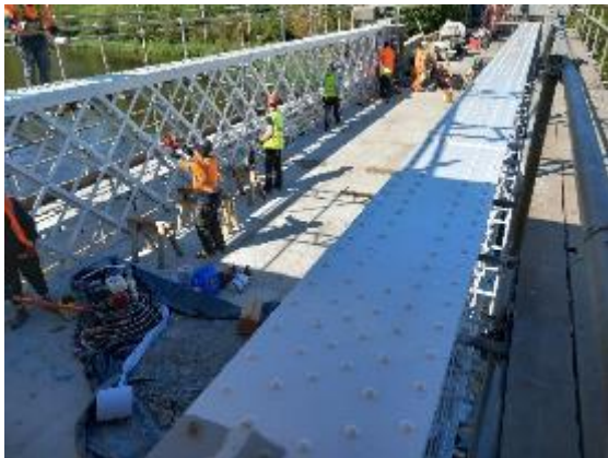
Bridge Final Steel Painting touching up and scaffolding stripped Bridge Northside
