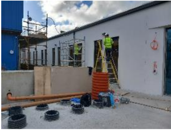
Block N North Elevation Final Rendering application and trimming around shadow gaps on windows.
