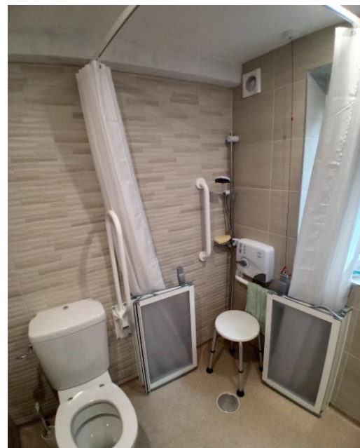
Bathroom Adaptation completed in in April in Dundalk with assistance of a Housing Adaptation Grant
