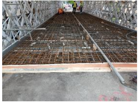
Bridge Deck Steel Reinforcement
