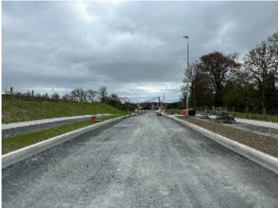
Works north of Lis na Dara
