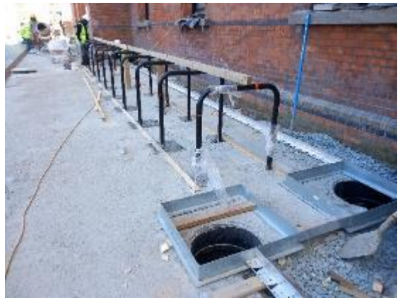
Block C Bicycle Stands to South elevation of Block (Area still to be paved)
