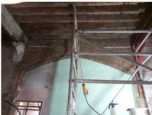
Block C Arch reinforcing
