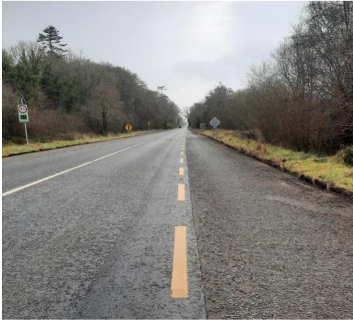
Road resurfacing works at Bellurgan
