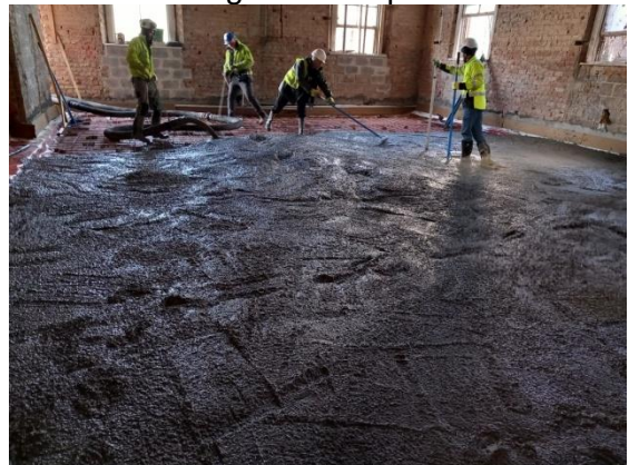
Block C Community Services Building –Floor pour
