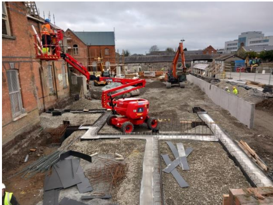
Block N Eastside Ground Beams
