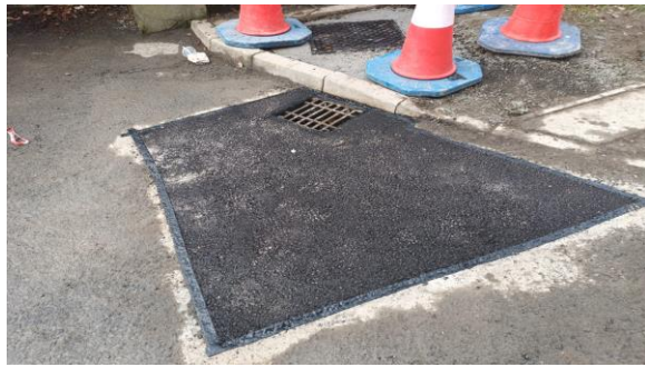
New gully & manhole in Tinure
