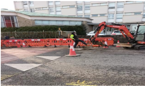
Ongoing works at Hardiman's Gardens
