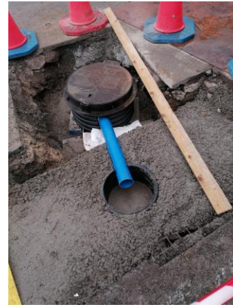
New Chamber joining existing culvert to existing 450mm diameter concrete pipe
