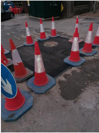
Completed works at new chamber over culvert
