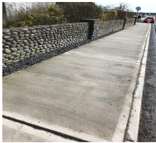
Renewed footpath at Annagassan.
