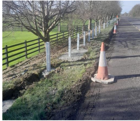
Installation of Crash Barriers on N53
