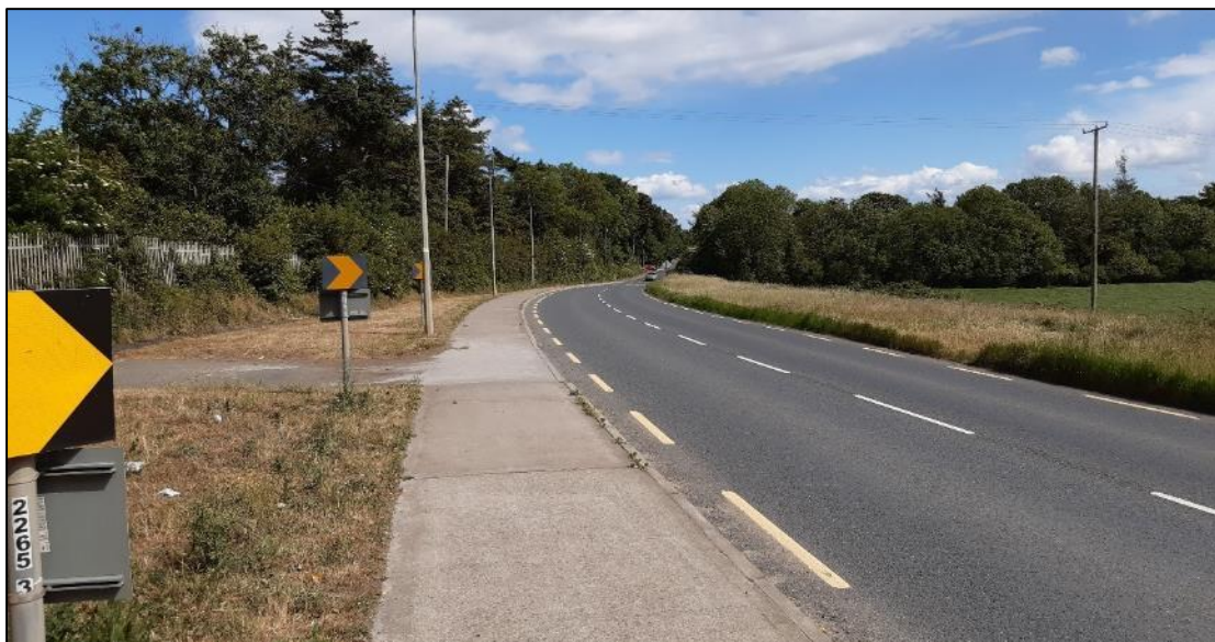
Figure 4.8 Footpath provision on N52
