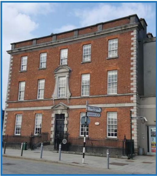
PHOTO 3.19 Exterior of Barlow House, Narrow West Street
