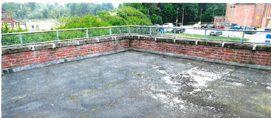
Current condition of roof 2.
